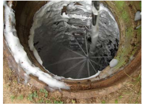
Root Control Program: manhole being treated
