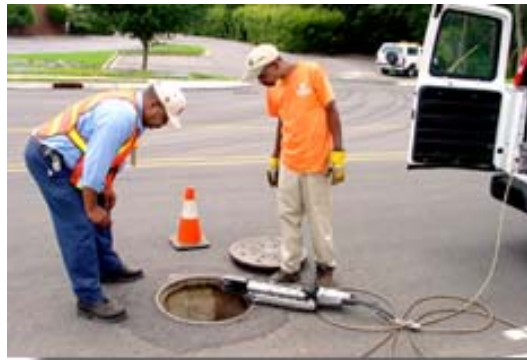
Crews use robotic cameras to check wastewater pipes
