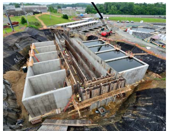
Filter expansion at McAlpine WWTP
