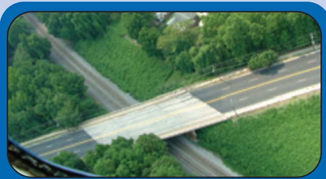
CATS is coordinating with the North Carolina Railroad to run the Blue Line Extension in a portion of their right-of-way.
