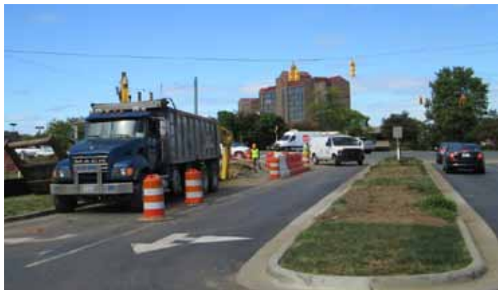
Watch for lane closures as construction gears up.
