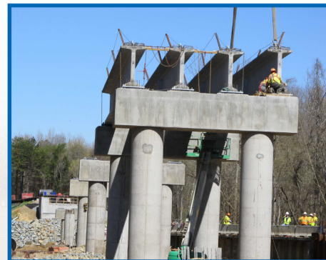
Light rail bridge over Toby Creek
