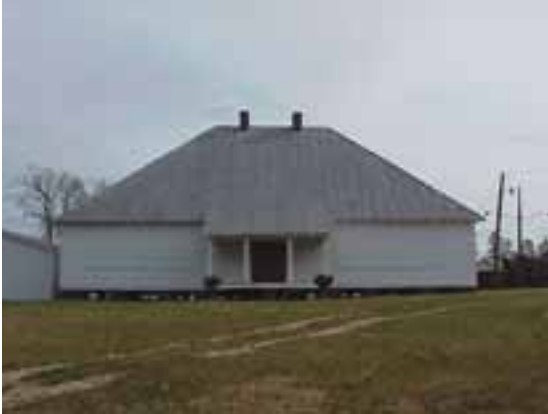
Mallard Creek Community Schoolhouse
