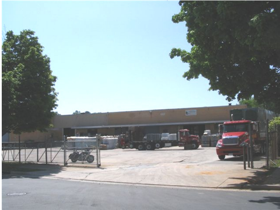
Plate 48. Standard Chemical Products Plant, Rear Warehouse and Loading Docks, Looking South.
