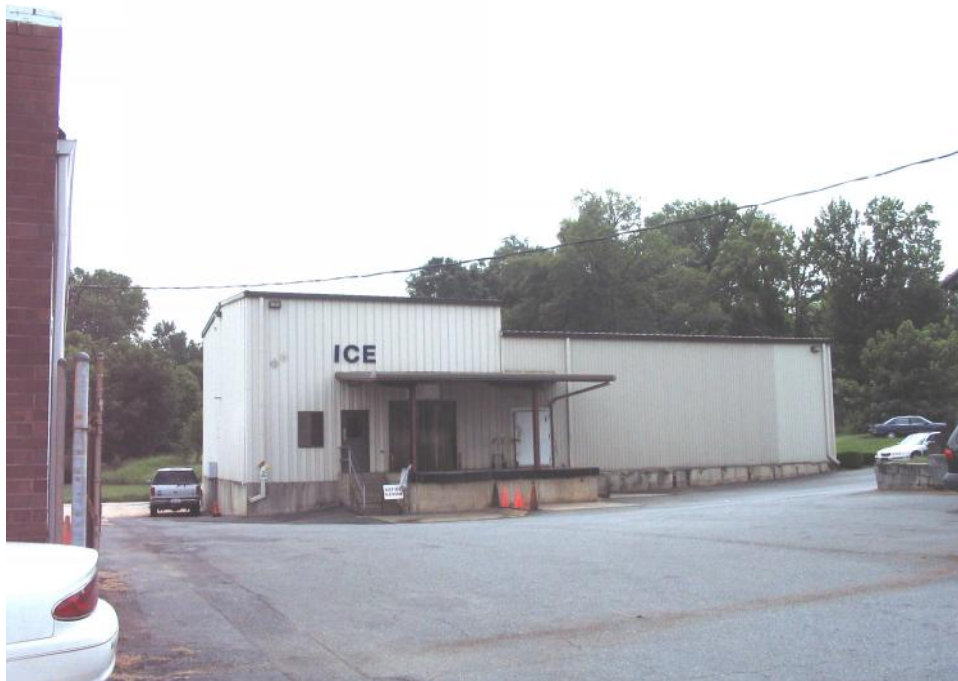
Plate 41. Herrin Brothers Coal and Ice Company Complex, Modern Ice House, Looking East.
