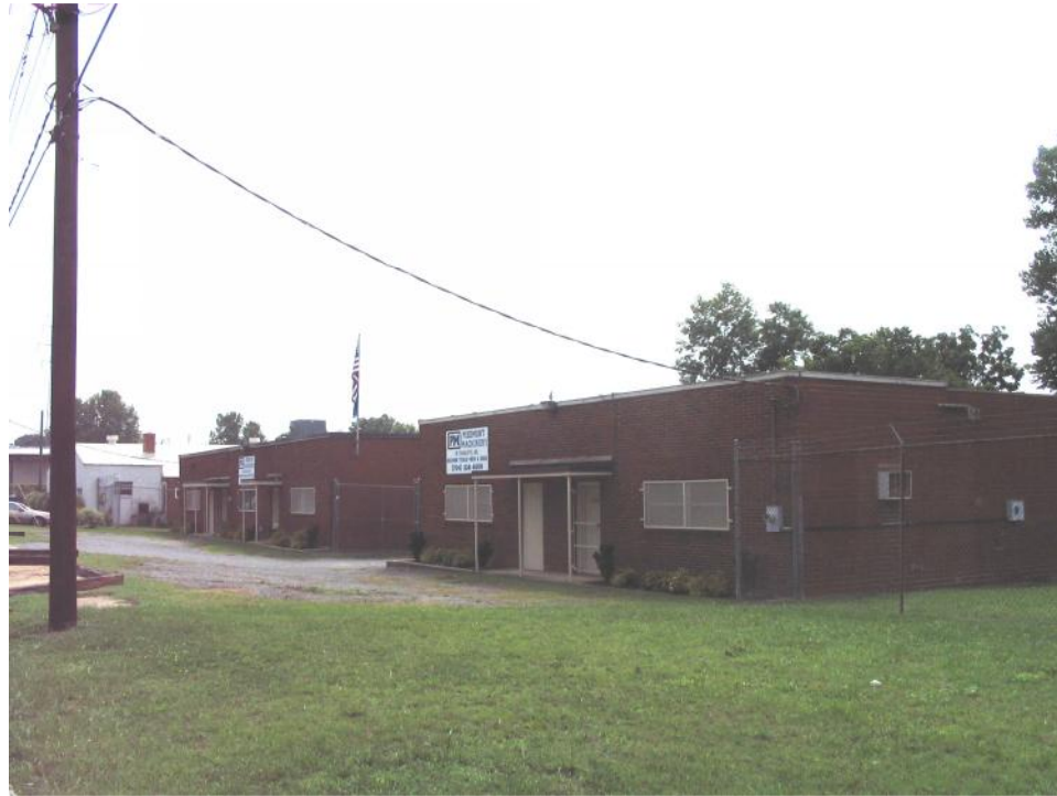
Machine Shop Complex (No. 28).
