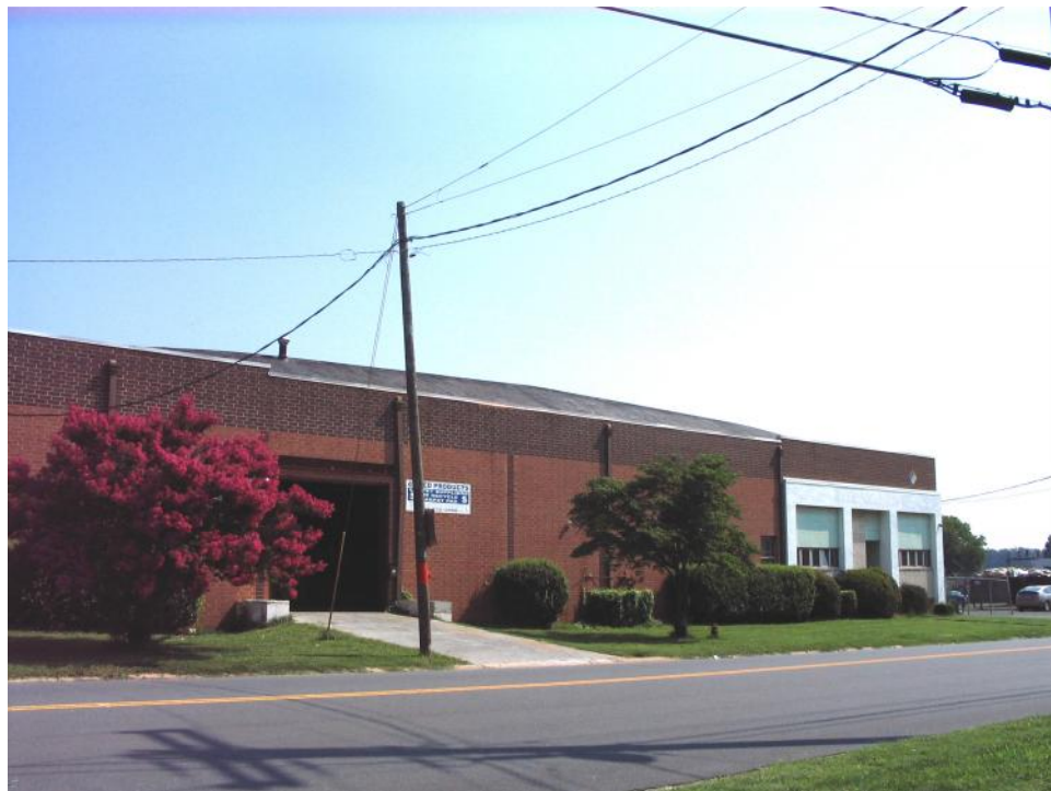
Industrial Building (No. 59).
