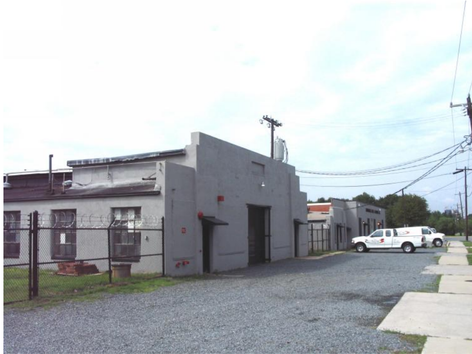
Machine Shop Complex (No. 18).
