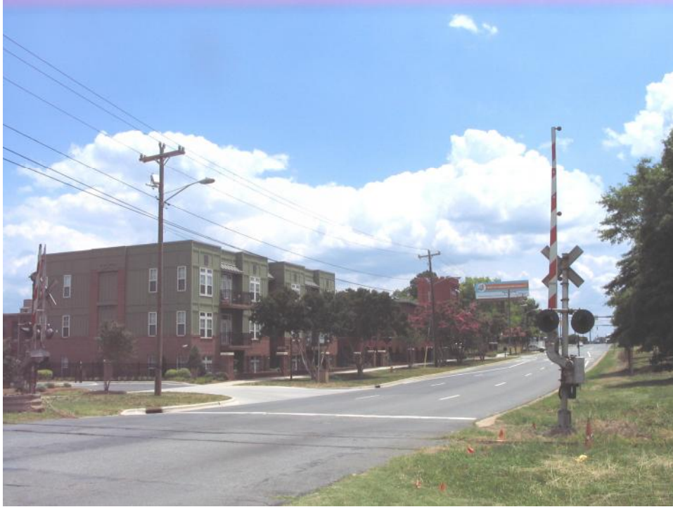
Plate 15. Orient Manufacturing Company/Chadwick-Hoskins No. 3, New Apartment Building, Looking East Along East 12 th Street Across Railroad Corridor.
