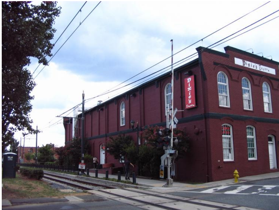
Plate 2. Philip Carey Company Warehouse, Façade and Side (West) Elevation, Looking Northeast Across Existing LYNX Blue Line.
