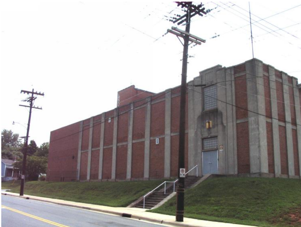
Plate 21. Chadbourn Hosiery Mills, Front (West) Elevation, Looking Northeast From North Brevard Street.
