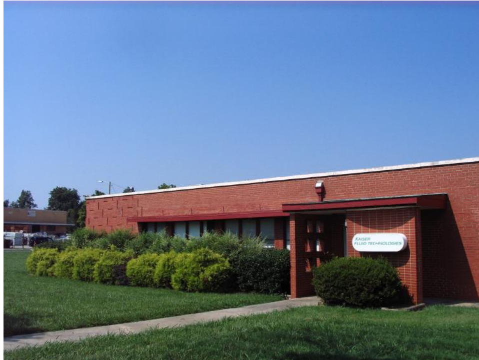
Kaiser Fluid Technologies Company Plant (No. 72), Front (East) Elevation of Office Section.
