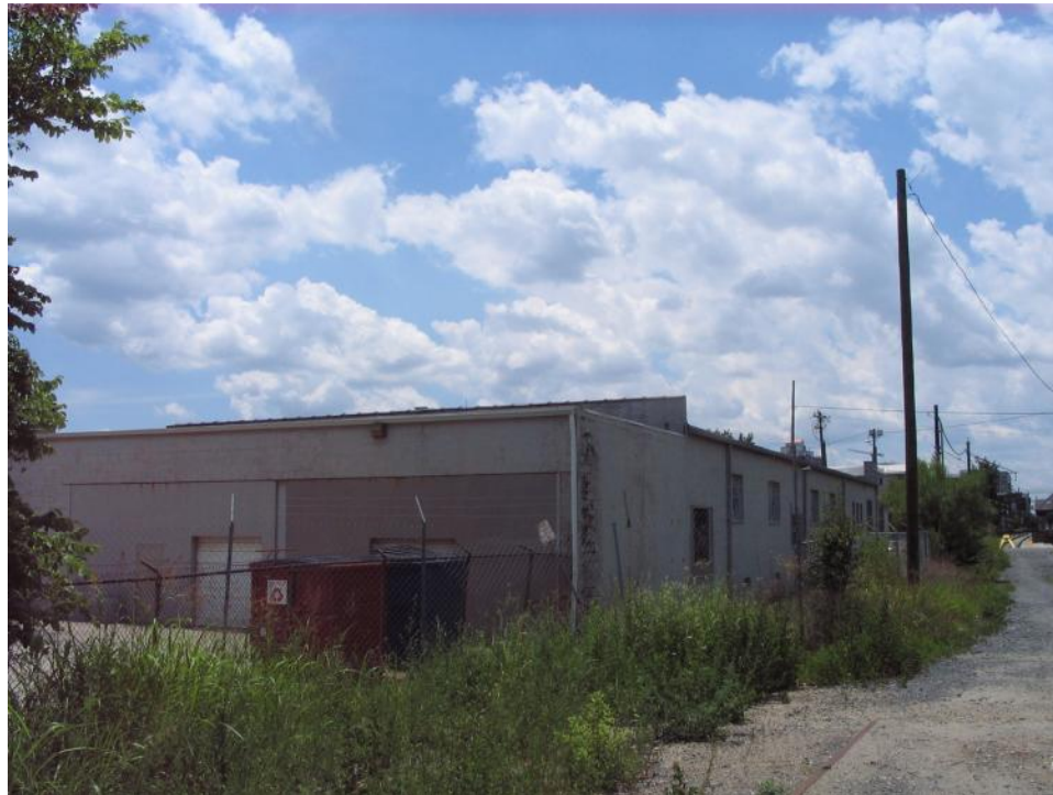
Warehouse (No. 3), Rear Elevation.
