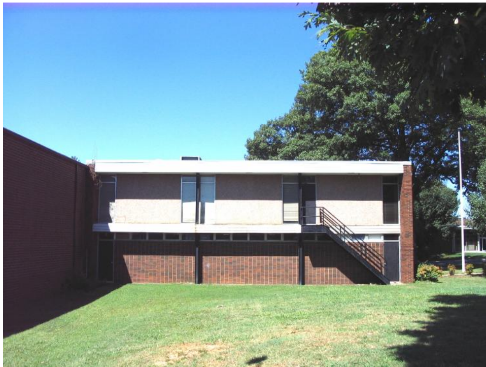
Truck Drivers Union (AFL No. 71) Hall (No. 76), East Elevation, Looking West, Auditorium Addition on Left.
