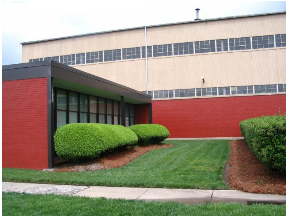
Plate 56. Republic Steel Corporation Plant, Office, South Elevation and Warehouse, West Elevation, Looking East.
