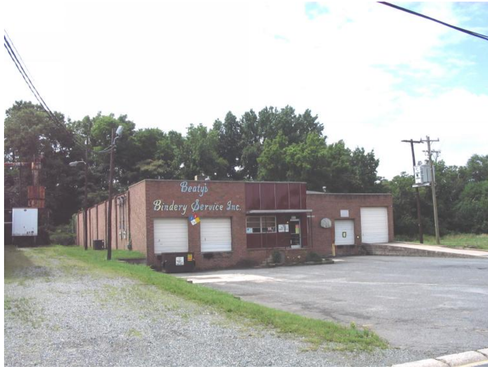
Industrial Building (No. 37).
