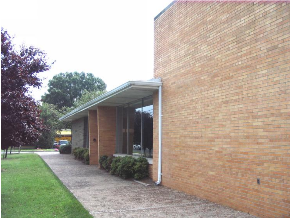
Plate 82. General Motors Corporation Training Center, Office and Auditorium, Façade (North Elevation), Looking Northeast.
