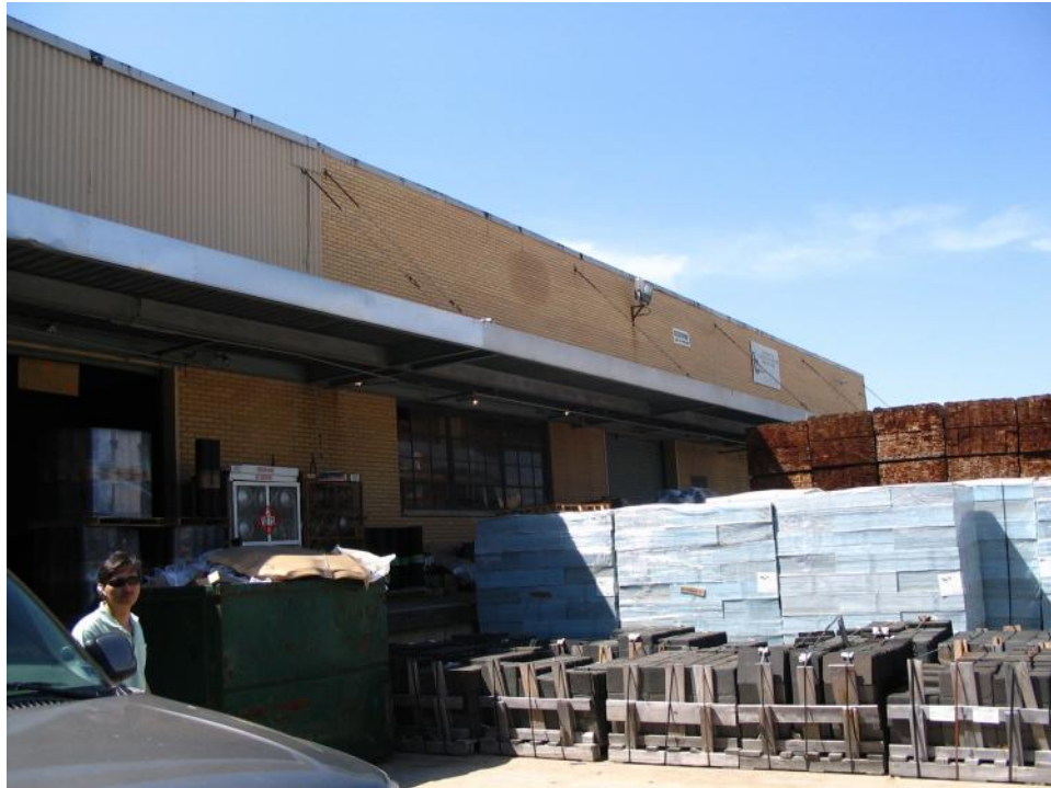
Plate 49. Standard Chemical Products Plant, Rear Warehouse and Loading Dock, North Elevation, Looking Southwest.
