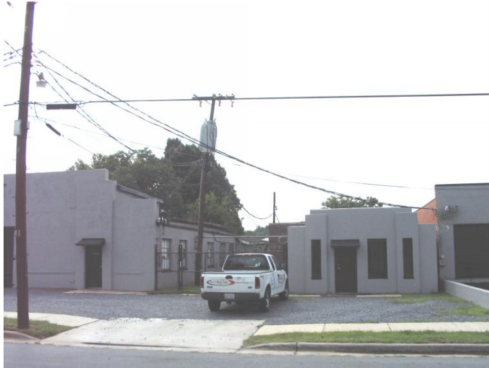
Machine Shop Complex (No. 18).
