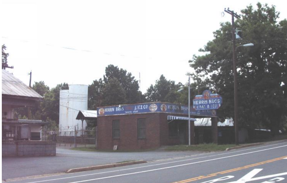
Plate 37. Herrin Brothers Coal and Ice Company Complex, Office (Right), Ice House (Left) and Oil Tank (Background), Looking Southeast.
