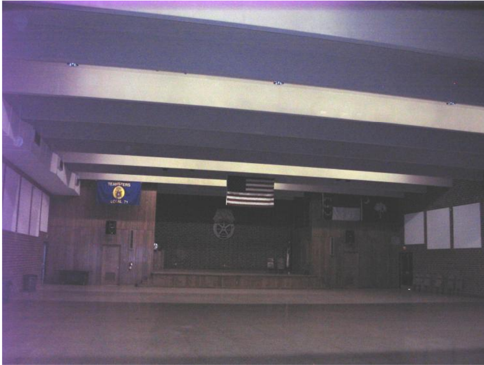
Truck Drivers Union (AFL No. 71) Hall (No. 76), Interior, Auditorium Addition.
