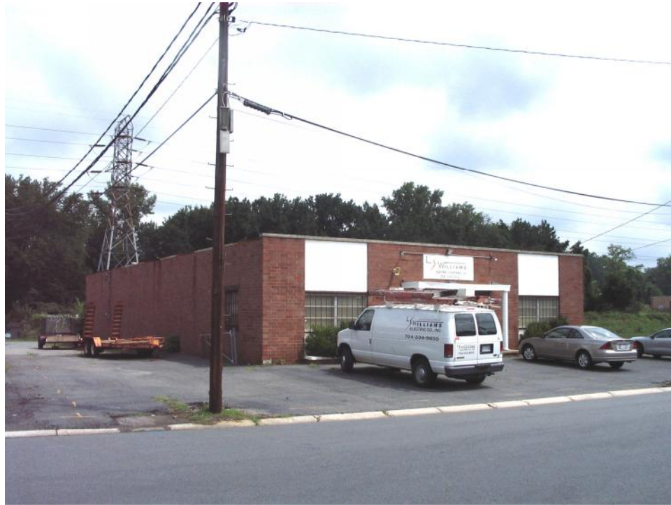
Industrial Building (No. 45).
