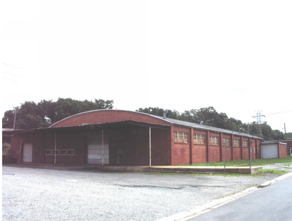
Industrial Building (No. 48), Rear (West) and Side (South) Elevations.
