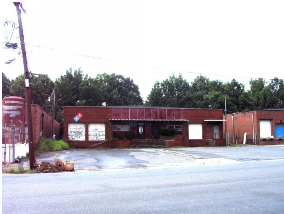
Industrial Building (No. 42).
