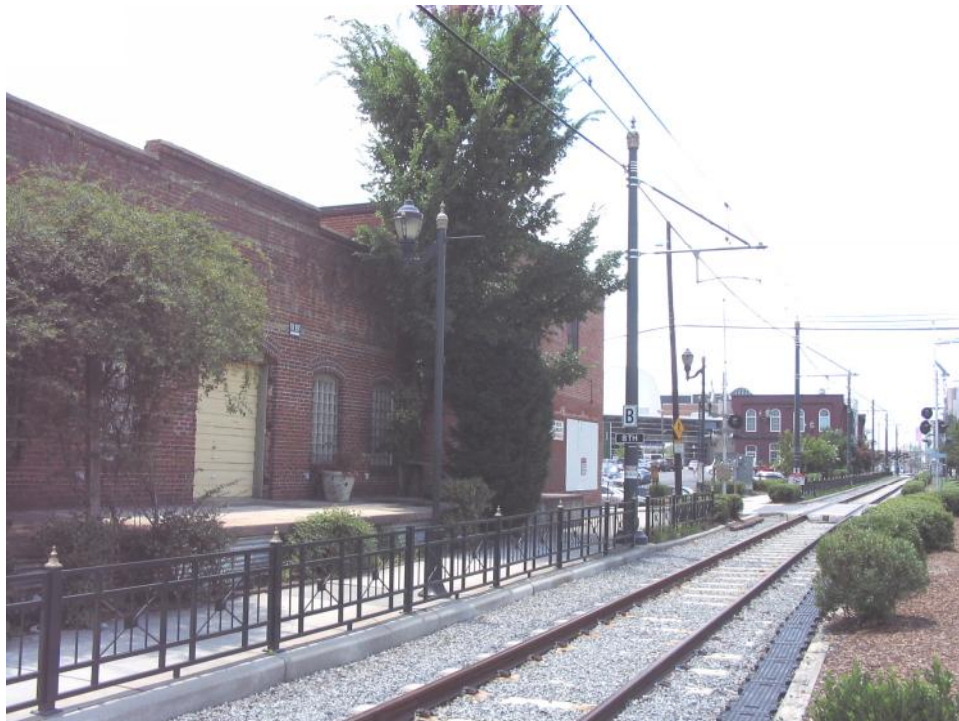
Plate 8. McNeil Paper Company Warehouse Complex, 305-307 East 8 th Street on Left, Looking South Along Existing LYNX Blue Line.
