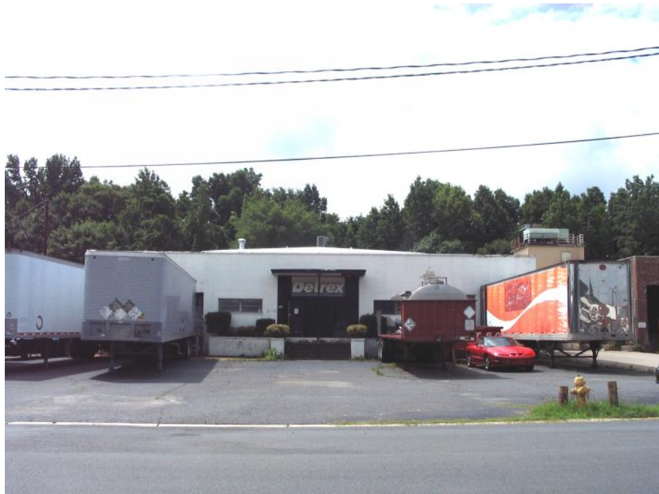
Industrial Building (No. 40).
