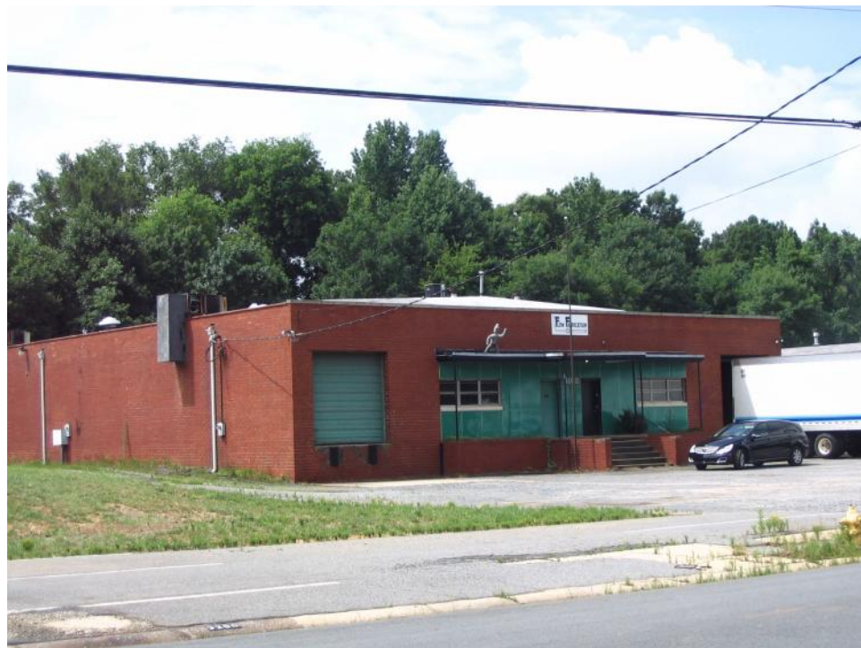
Industrial Building (No. 38).
