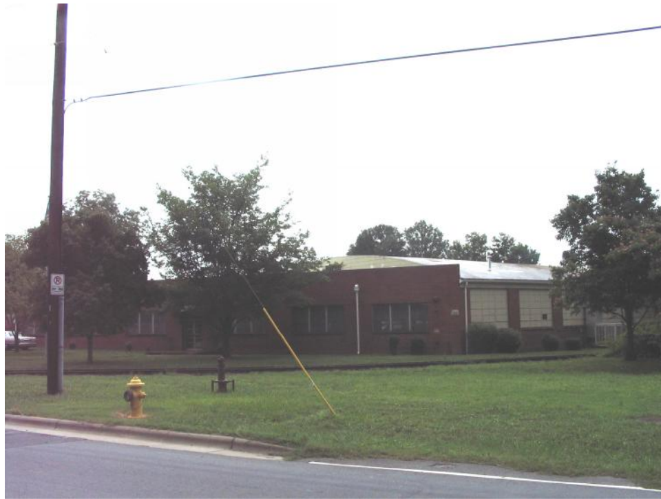
Industrial Building (No. 30).
