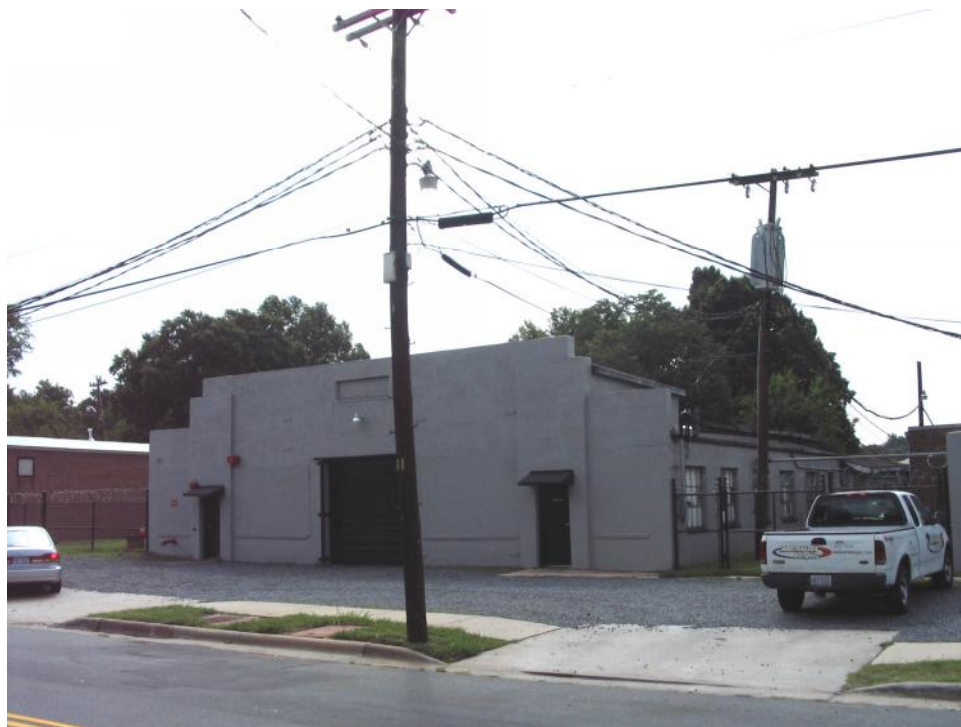
Machine Shop Complex (No. 18).
