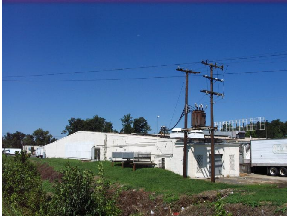
Plate 67. Park-n-Shop Supermart, Rear (South) Elevation, Looking Northwest.
