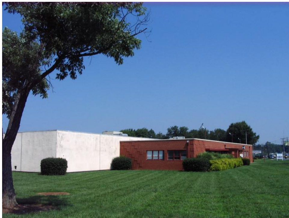
Kaiser Fluid Technologies Company Plant (No. 72).
