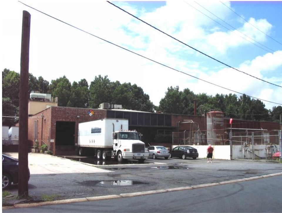
Industrial Building (No. 41).
