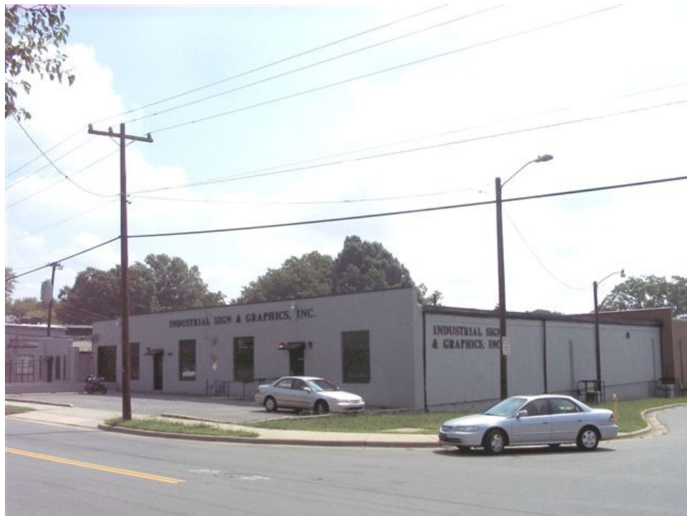
Industrial Building (No. 17).
