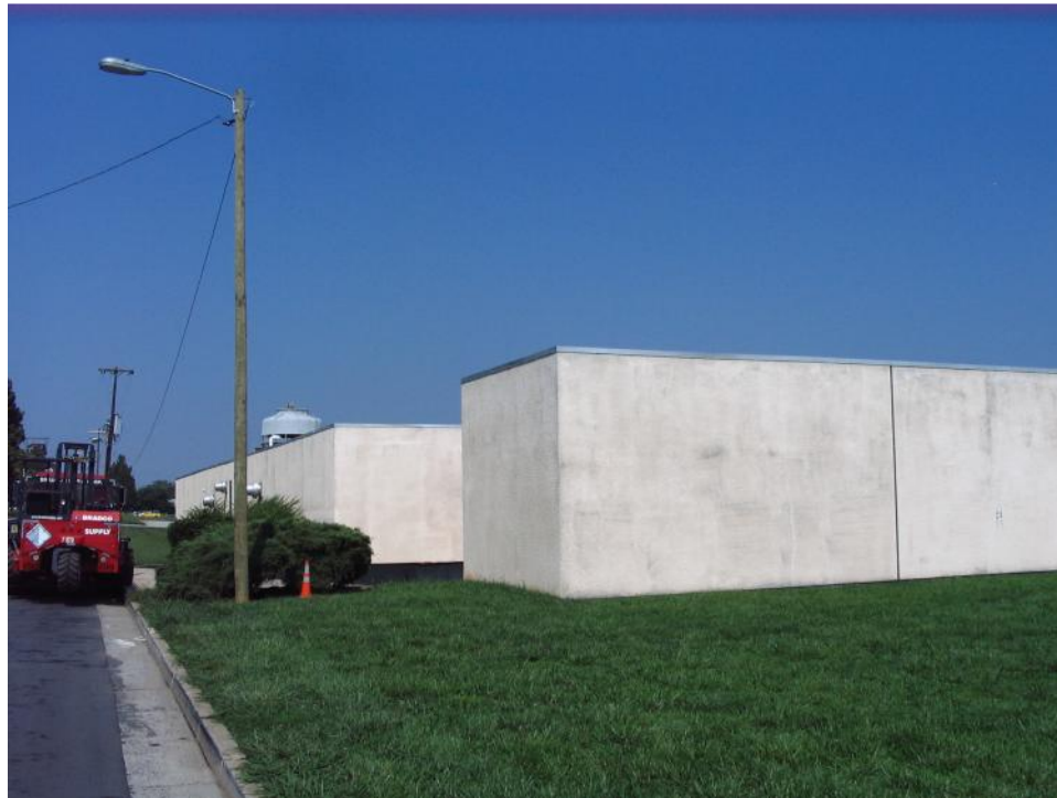
Kaiser Fluid Technologies Company Building (No. 72), Rear Manufacturing and Warehousing Wings, Looking Northwest.
