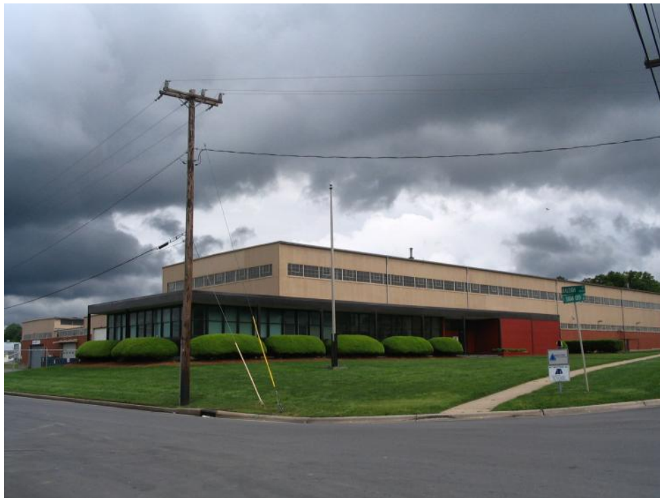
Plate 53. Republic Steel Corporation Plant, Office and Warehouse, Looking Southeast From Sugar Creek Road.
