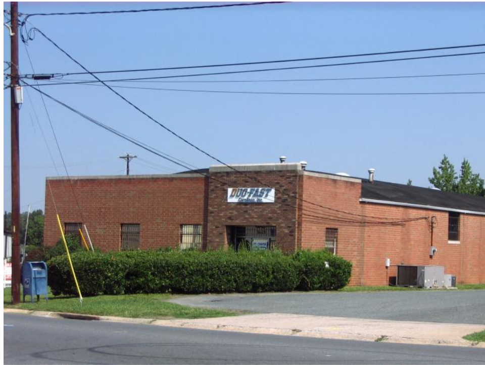
Industrial Building (No. 54).
