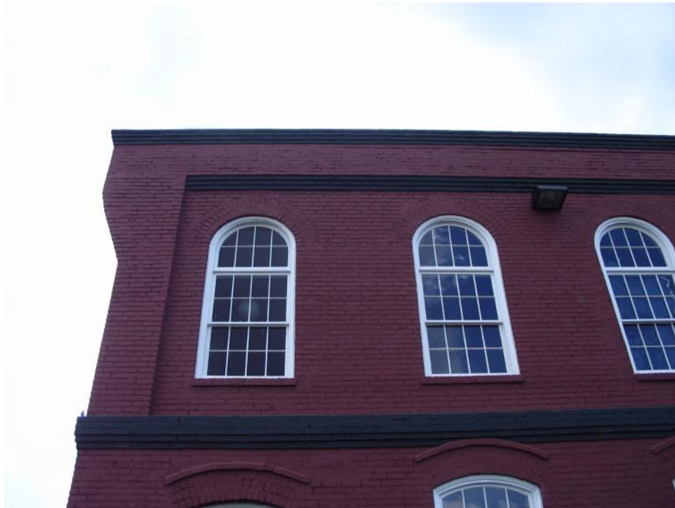
Plate 5. Philip Carey Company Warehouse, Detail of Windows and Brickwork.
