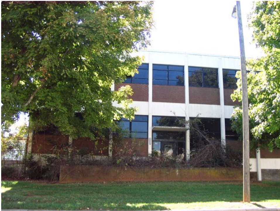
Plate 51. Standard Chemical Products Plant, 1967 Research Laboratory, Looking South.
