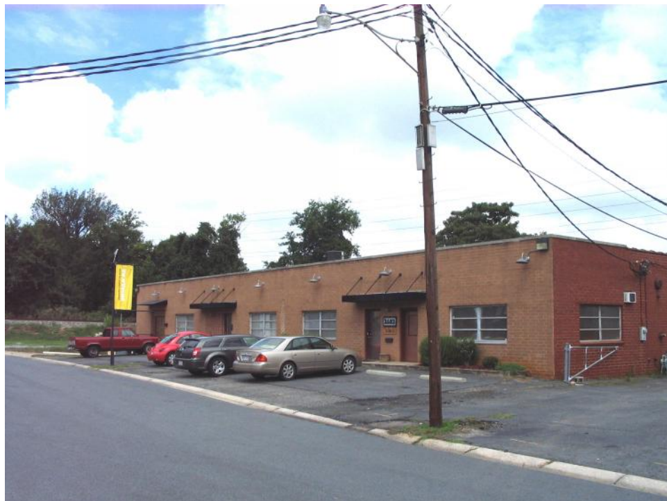
Industrial Building (No. 44).
