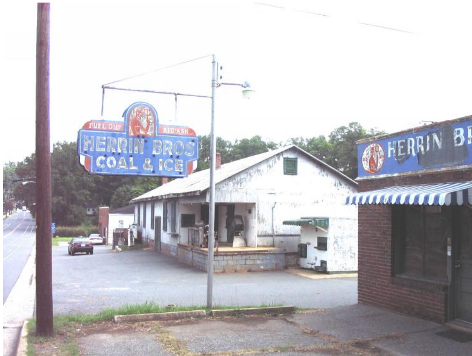
Plate 36. Herrin Brothers Coal and Ice Company Complex, Office (Right Foreground) and Ice House (Center), Looking North Along East 36 th Street.
