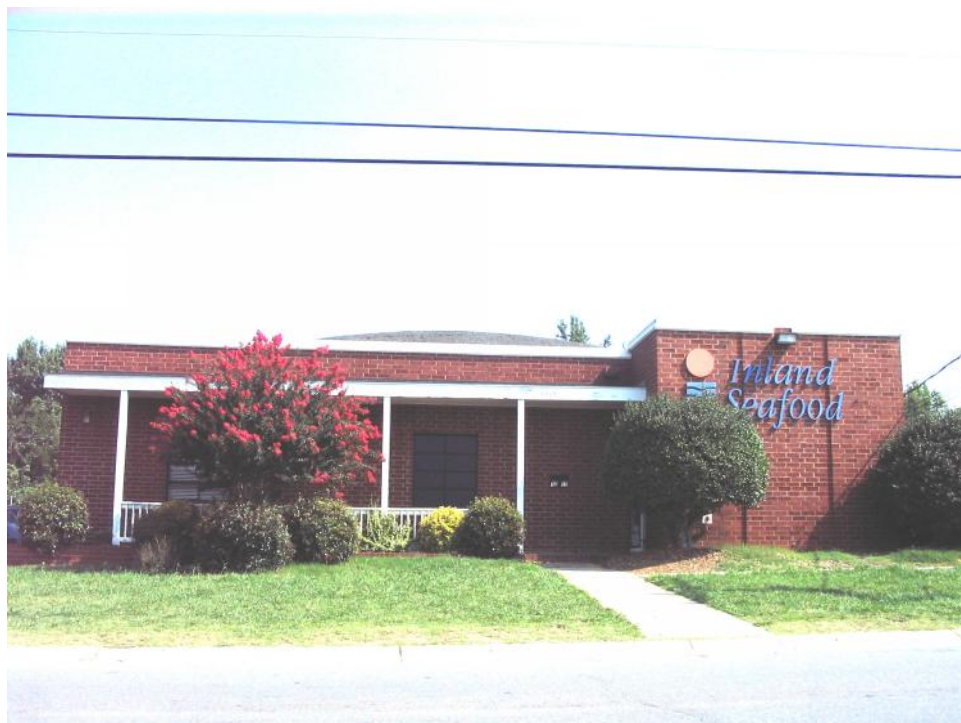
Industrial Building (No. 57), Front Elevation.
