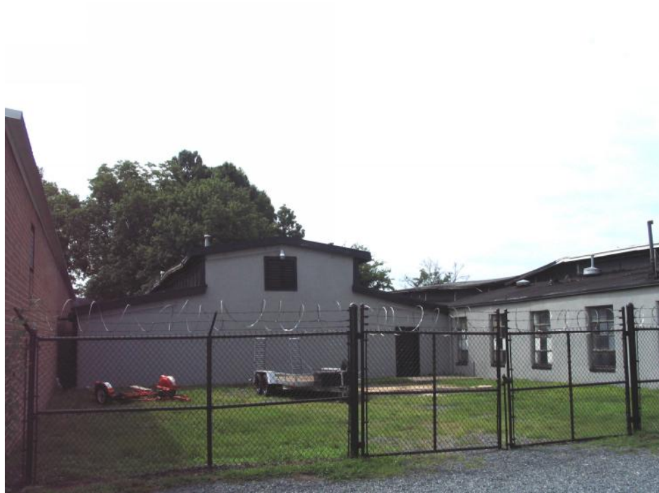
Machine Shop Complex (No. 18).
