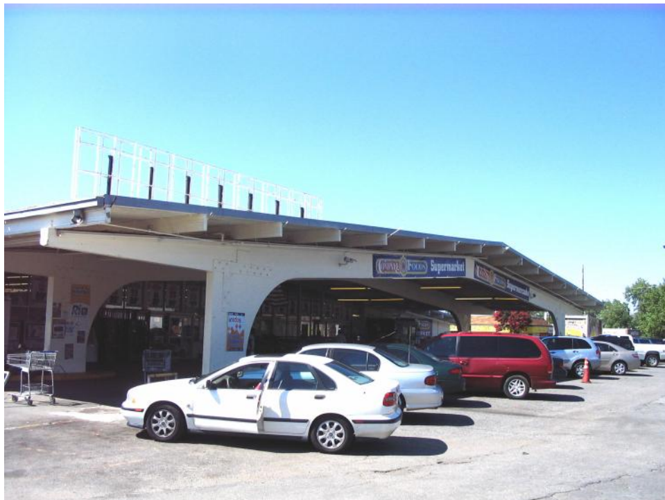
Plate 64. Park-n-Shop Supermart, Front (North) Elevation and Porte Cochere, Looking Southwest.
