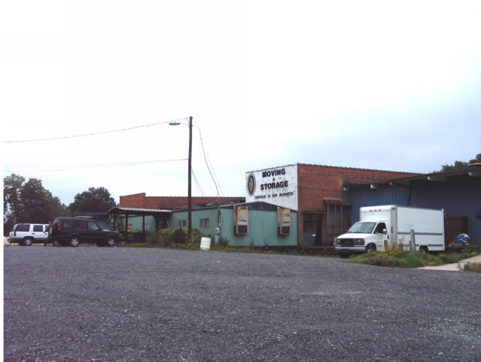
Merchants' Bonded Cotton Warehouse (No. 5).
