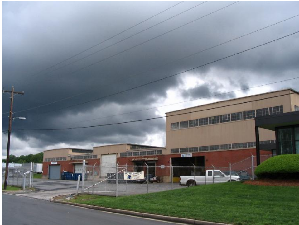
Plate 58. Republic Steel Corporation Plant, Fabricating and Warehousing Units, North Elevations, Looking Southeast.
