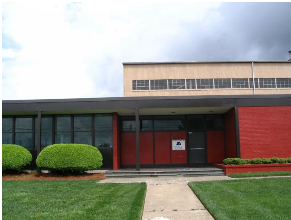
Plate 55. Republic Steel Corporation Plant, Office Entrance, Looking East.
