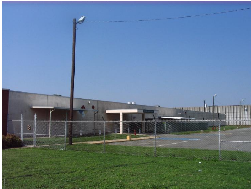
Kaiser Fluid Technologies Company Plant (No. 72), Rear Warehouse, Looking South.
