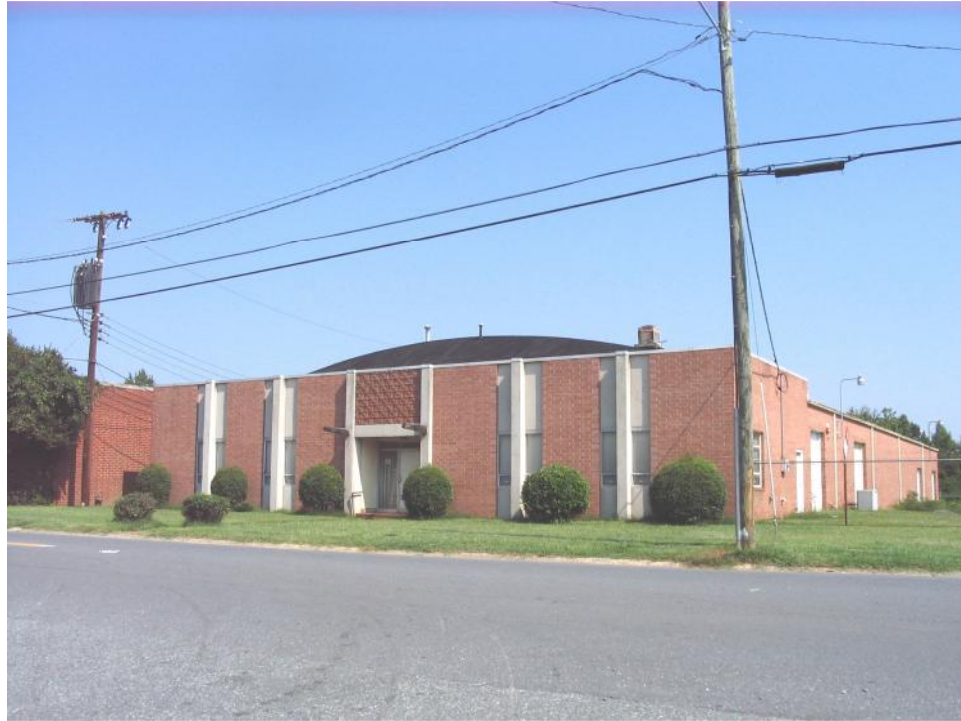
Industrial Building (No. 58).
