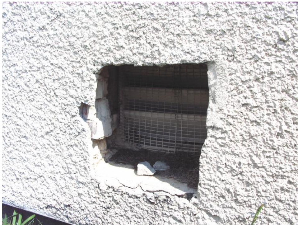
Kaiser Fluid Technologies Company Building (No. 72), Rear Warehouse, Detail of Stucco Covering Original Brick Veneer.
