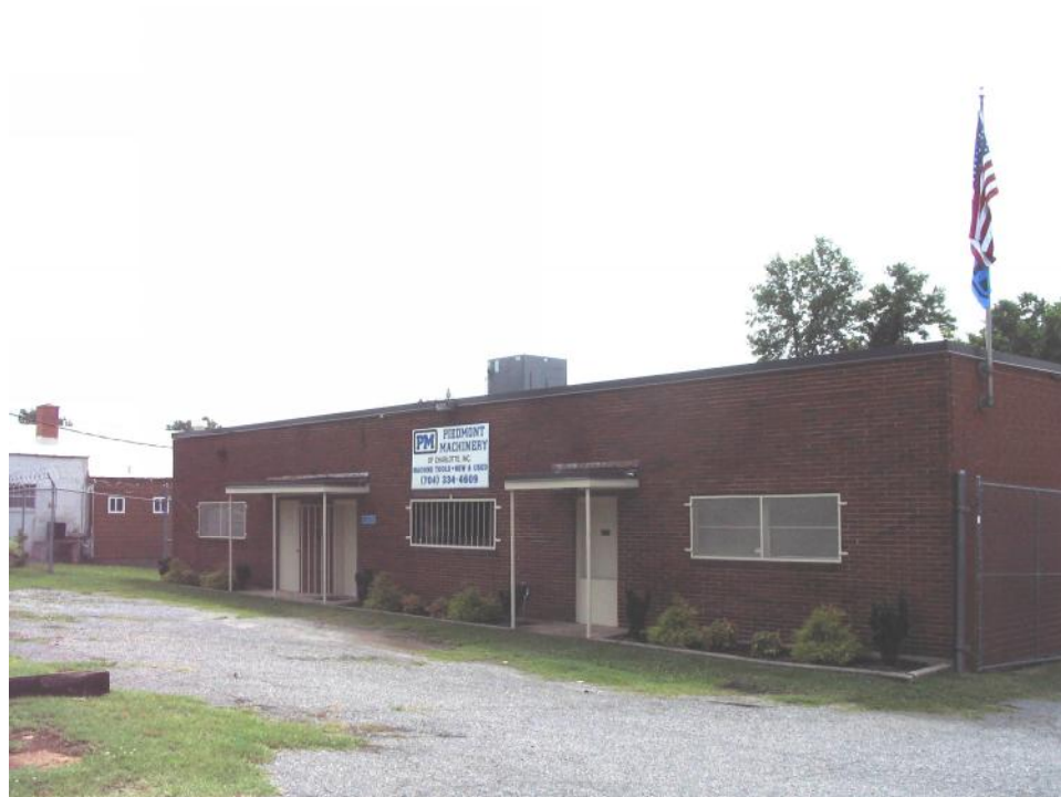
Machine Shop Complex (No. 28).
