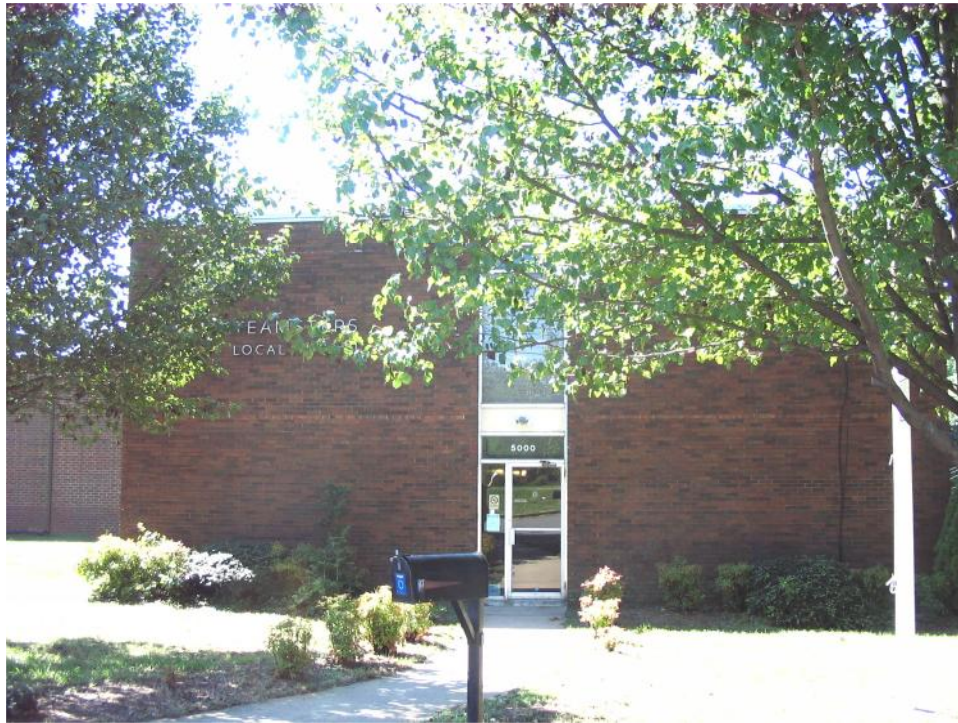
Truck Drivers Union (AFL No. 71) Hall (No. 76), North Elevation, Looking South.
