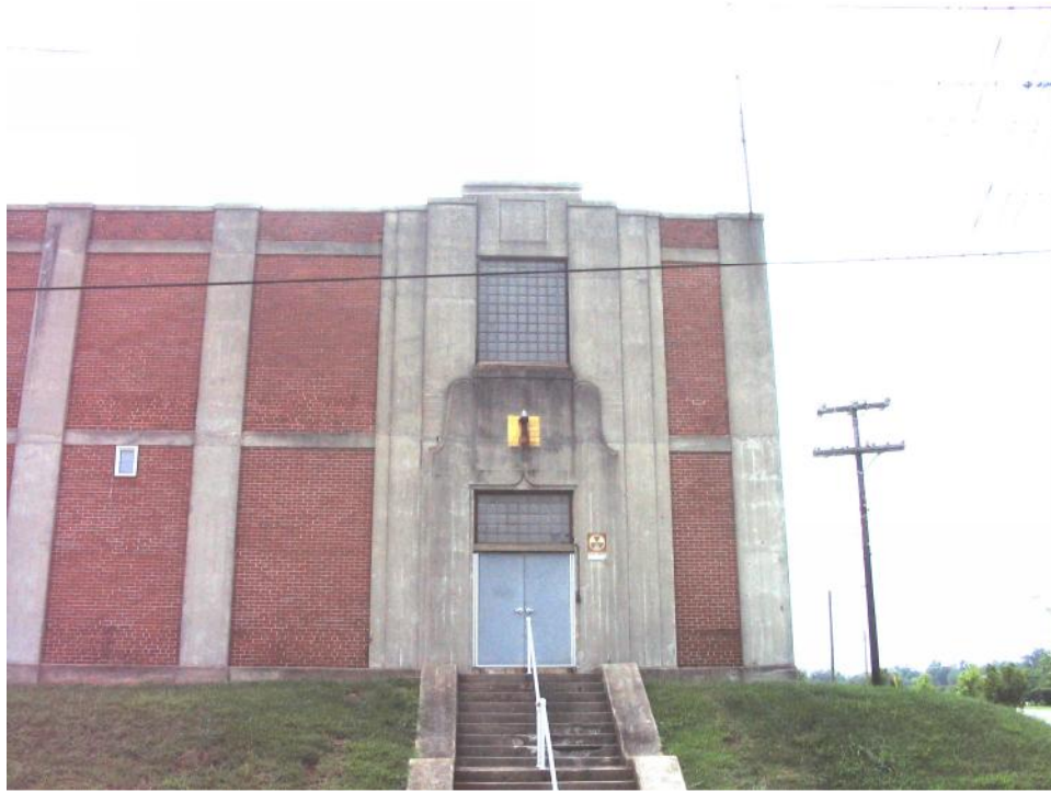
Plate 22. Chadbourn Hosiery Mills, Front (West) Elevation, Entrance.
