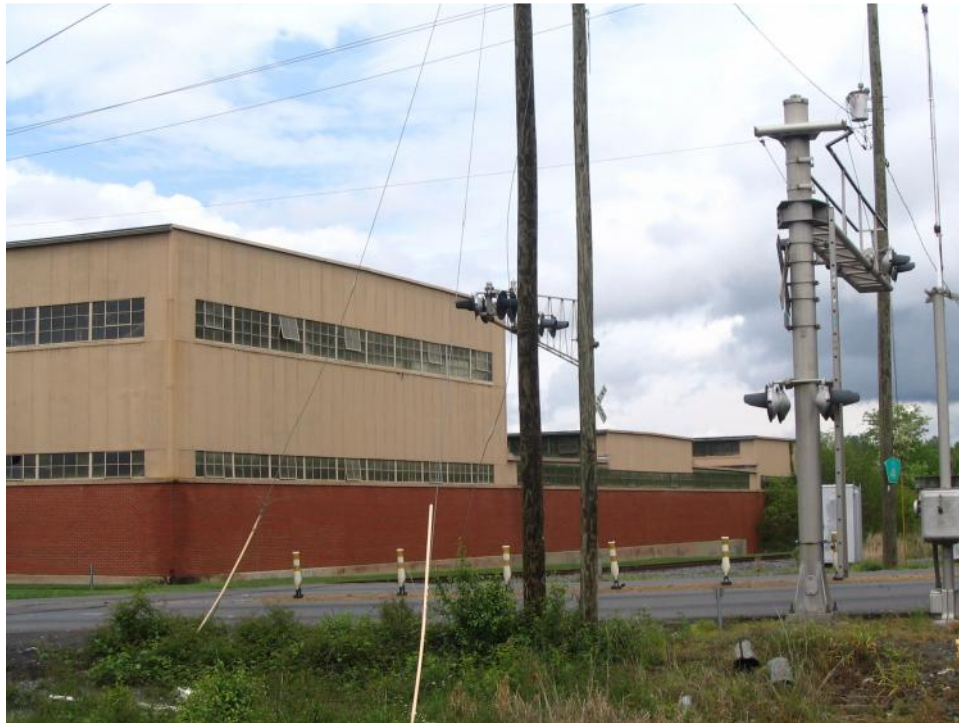
Plate 60. Republic Steel Corporation Plant, Fabricating and Warehousing Units, South Elevation, Looking Northeast From Railroad Corridor.
