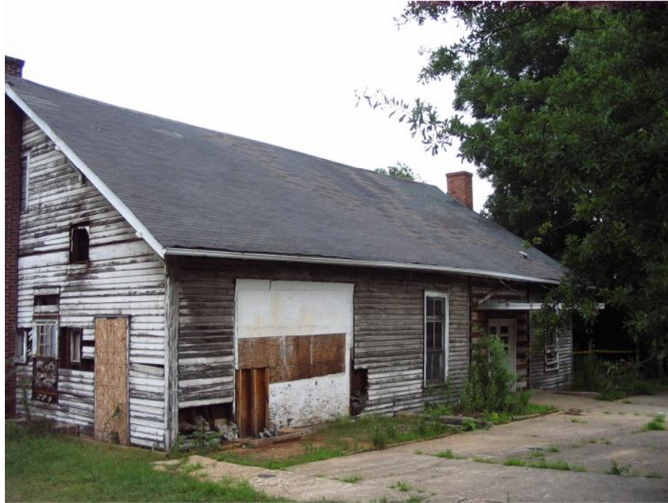
Storage Building (No. 6).
