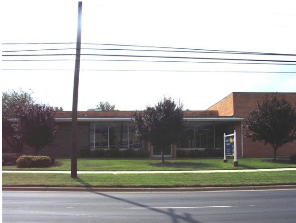
Plate 81. General Motors Corporation Training Center, Overall View, Office Façade (North Elevation), Looking Southeast.
