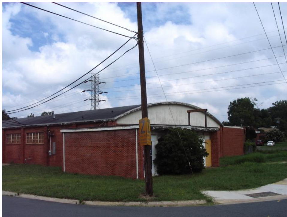
Industrial Building (No. 48).
