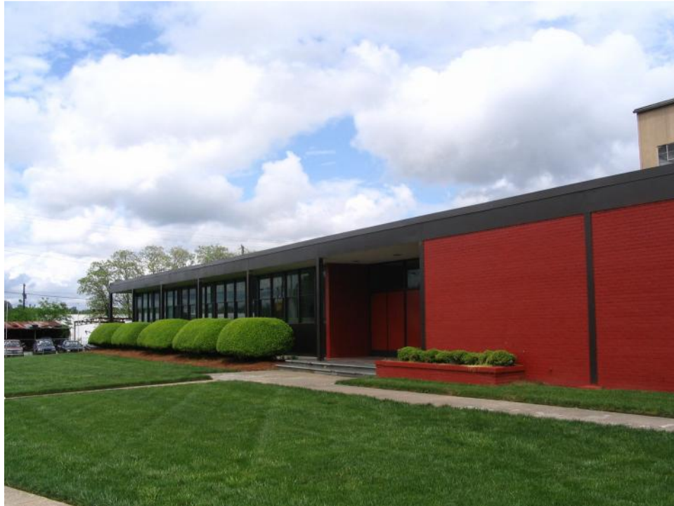
Plate 54. Republic Steel Corporation Plant, Office and Lawn, Looking North.
