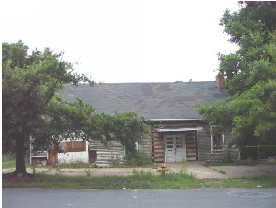
Storage Building (No. 6).
