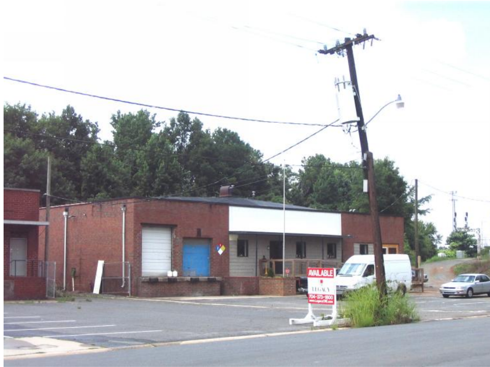
Industrial Building (No. 43).
