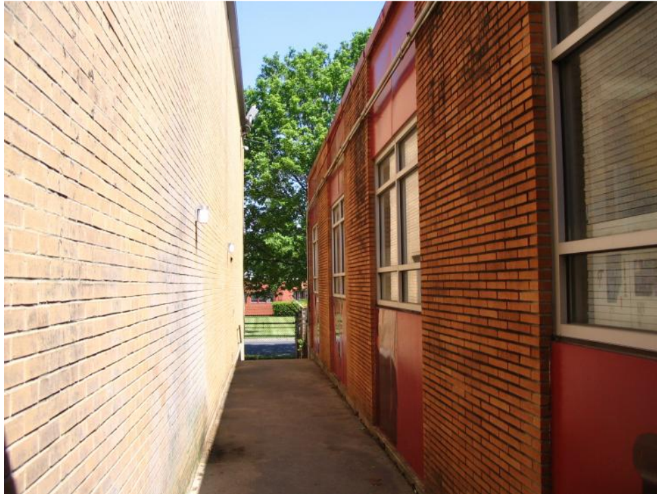
Plate 46. Standard Chemical Products Plant, Ramp Separating Office (Rear Elevation) and Warehouse, Looking North.
