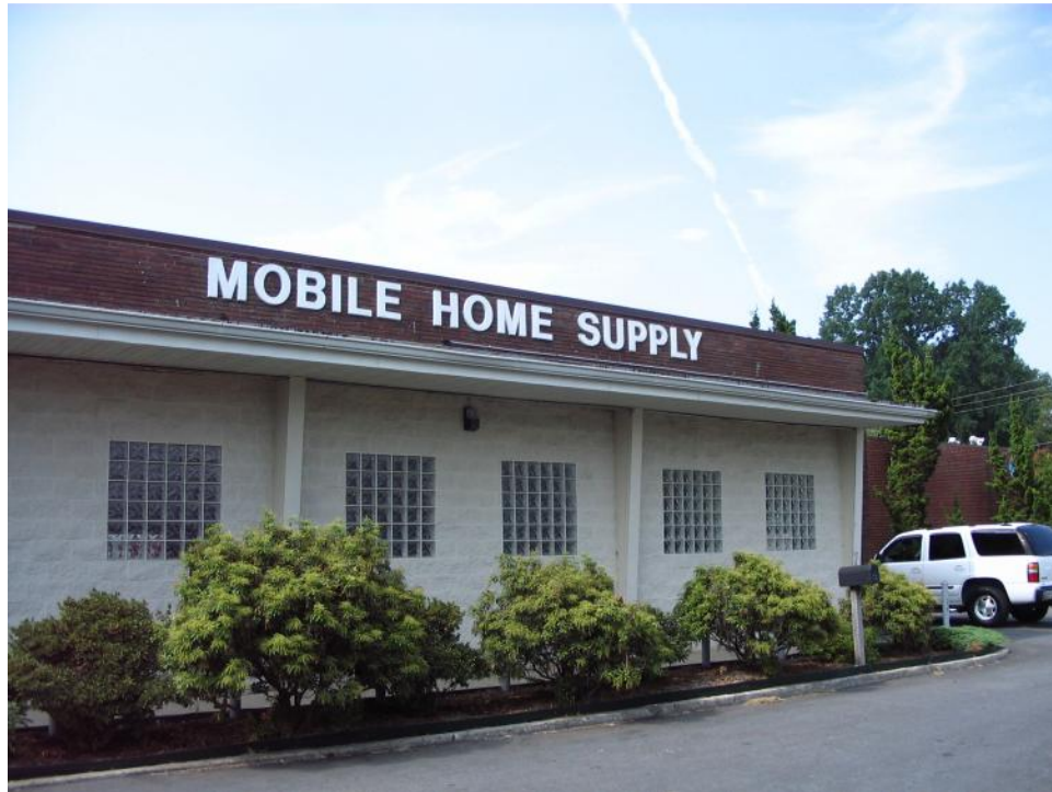
Mobile Home Supply Company Building (No. 75), Storefront Windows Infilled with Concrete Block and Glass Block.
