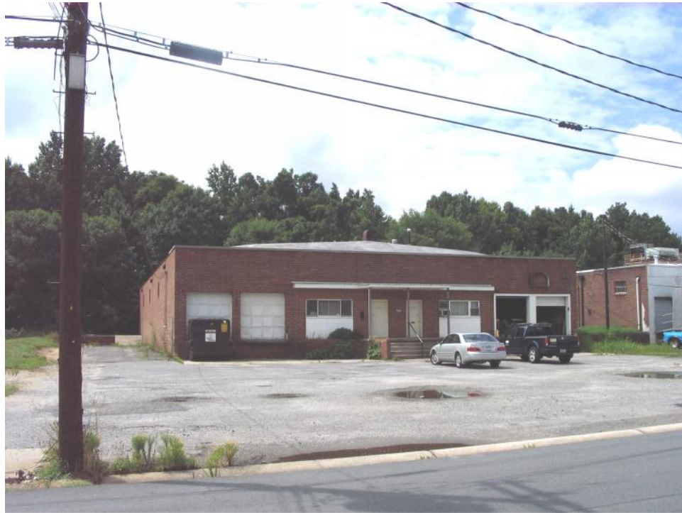
Industrial Building (No. 39).
