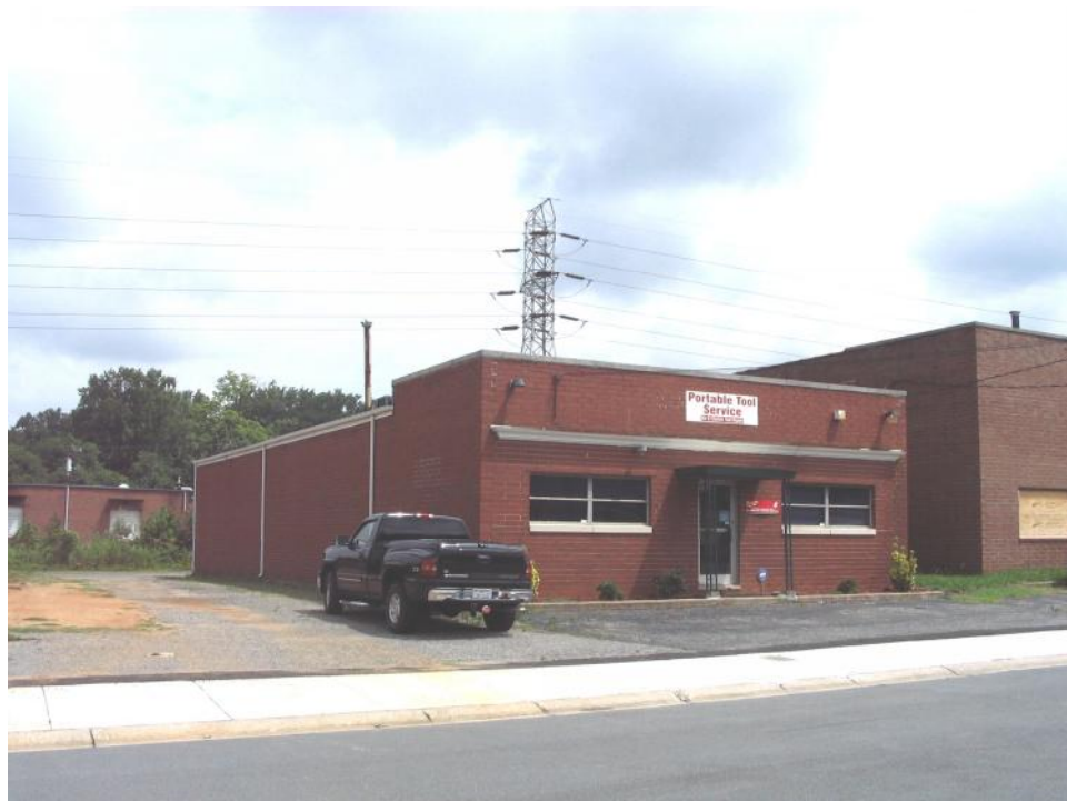
Industrial Building (No. 46).
