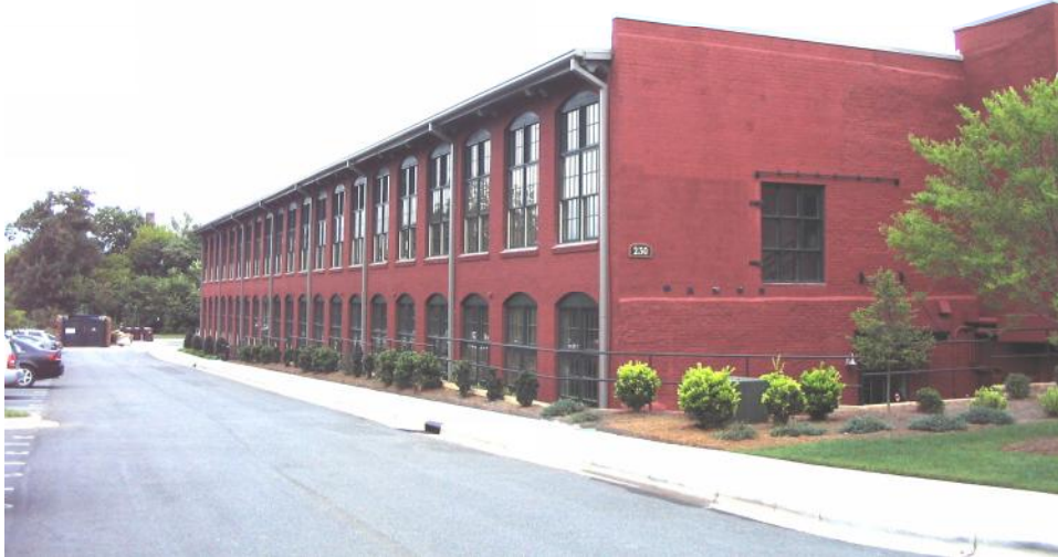
Plate 17. Orient Manufacturing Company/Chadwick-Hoskins No. 3, ca. 1911 Weaving Building, Looking East.
