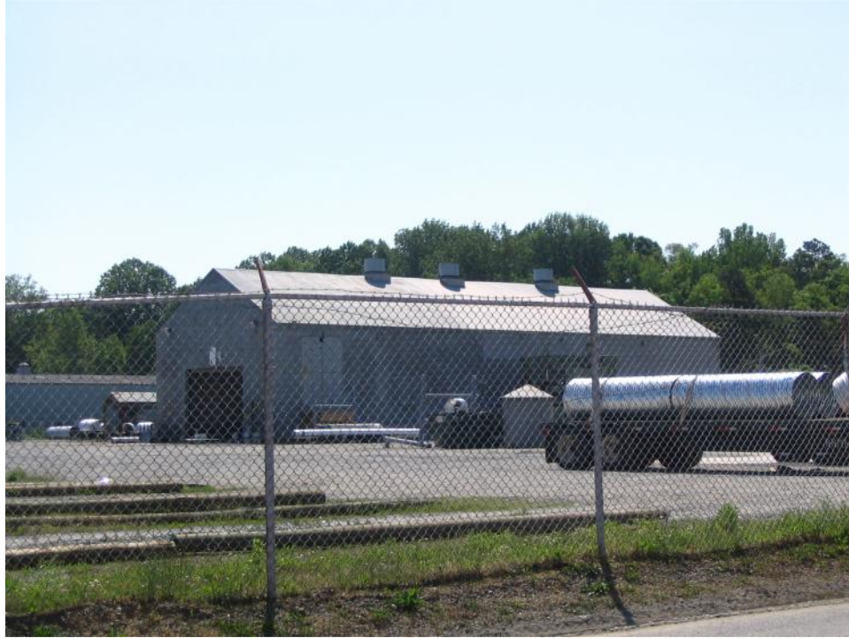
Plate 62. Republic Steel Corporation Plant, Pipe Fabrication Building at North End of Tract, Looking Southeast.
