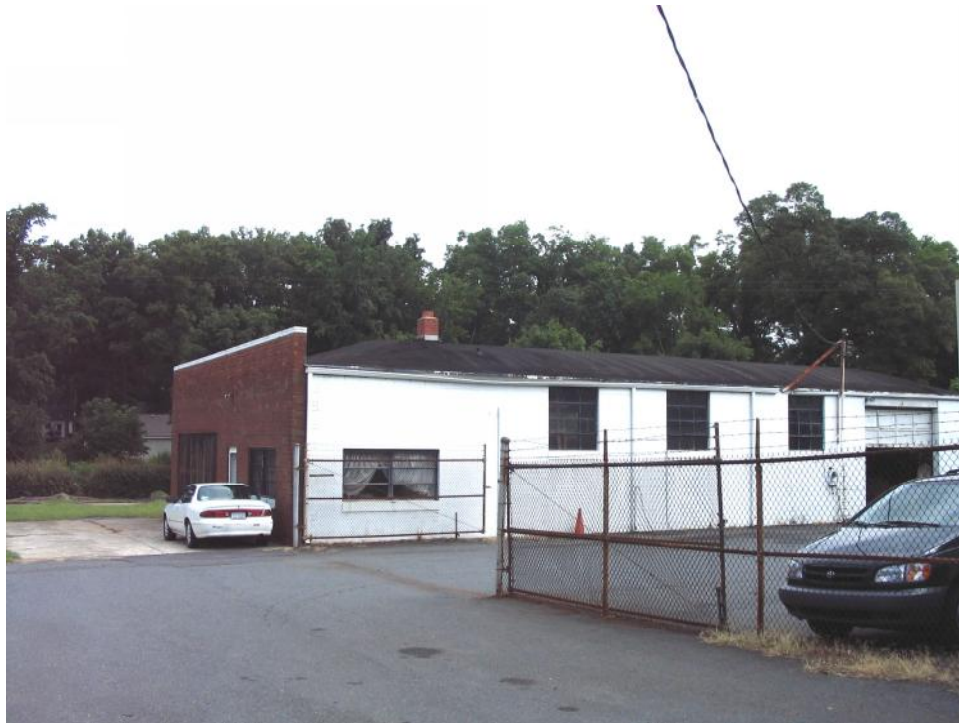
Plate 39. Herrin Brothers Coal and Ice Company Complex, Woodworking Shop/Garage, Looking North.
