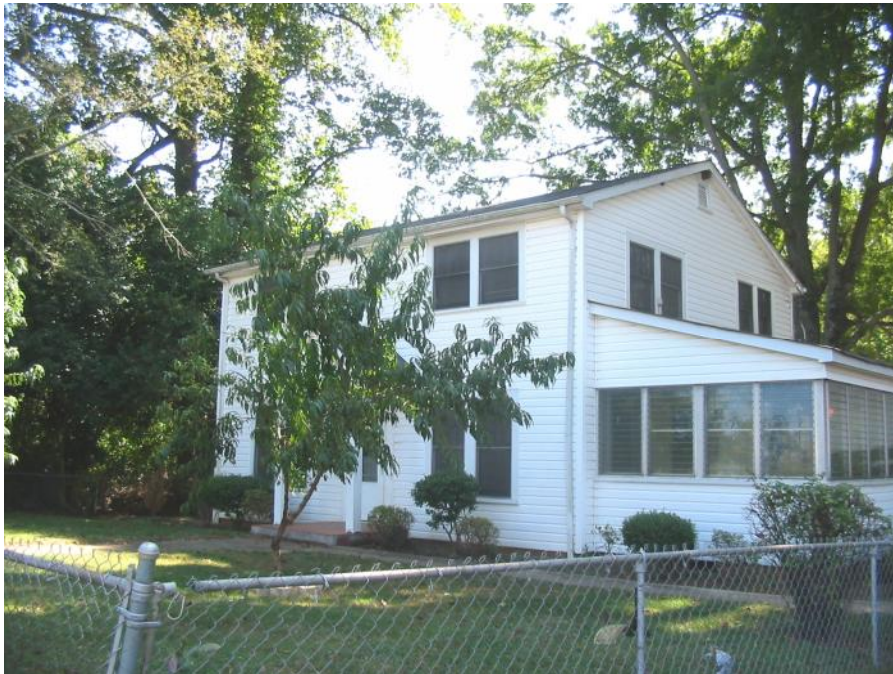
Plate 73. Elmore Trailer Sales and Trailer Park, Elmore House, Looking Southeast.
