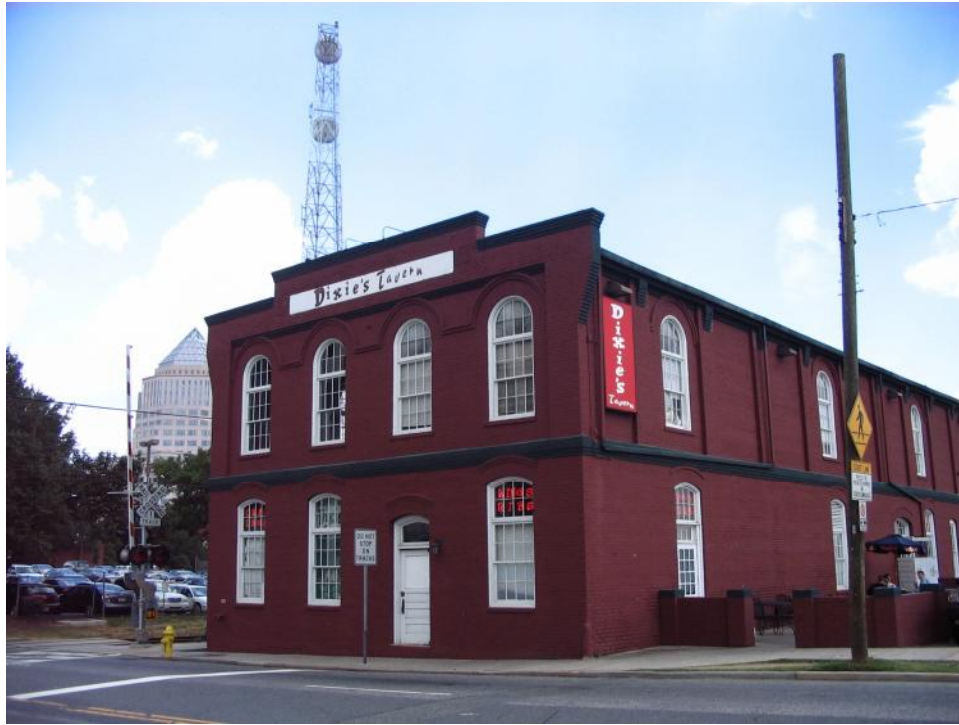
Plate 1. Philip Carey Company Warehouse, Façade and Side (East) Elevation, Looking Northwest.
