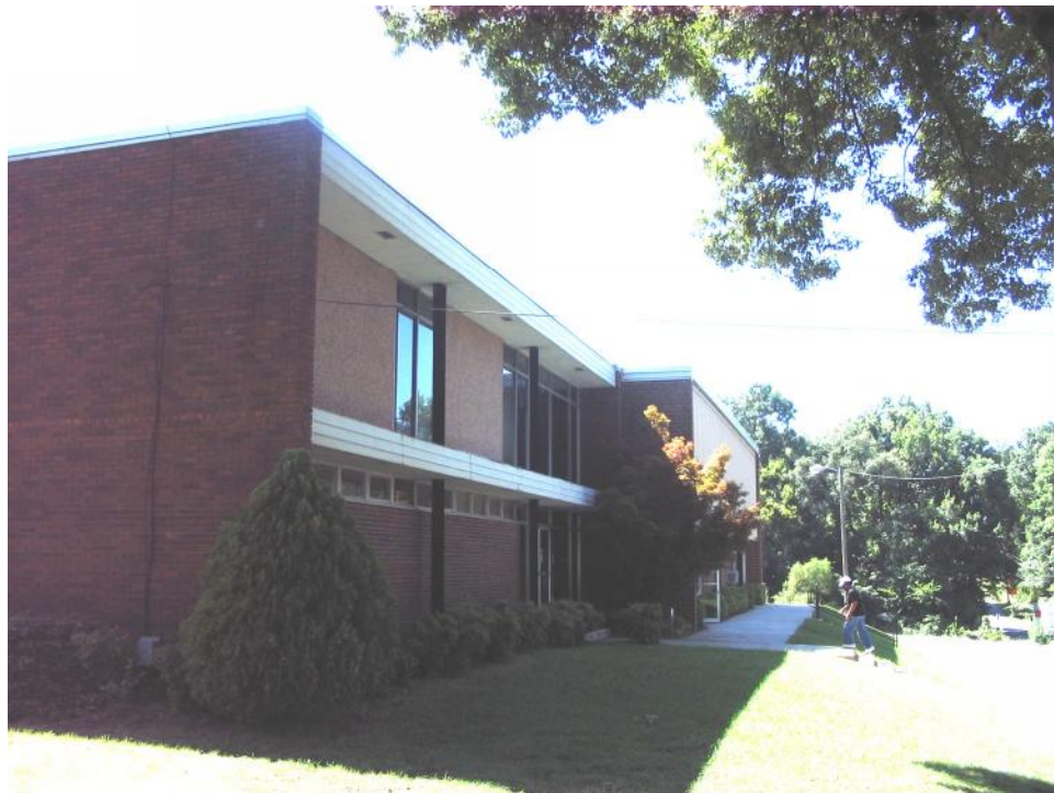
Truck Drivers Union (AFL No. 71) Hall (No. 76), Principal (West) Elevation, Looking South.
