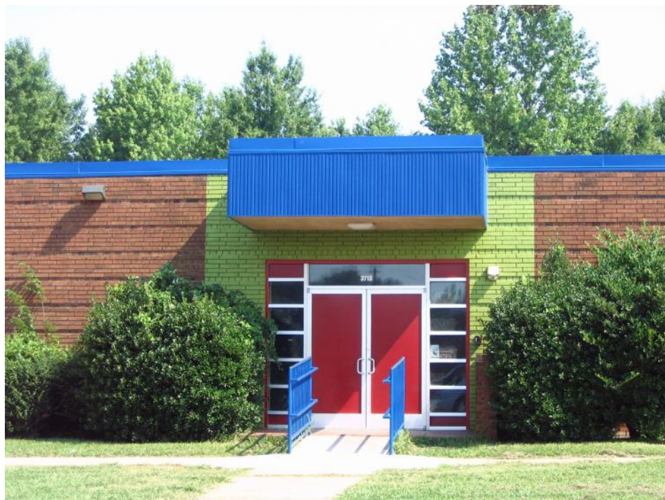
Industrial Building (No. 56), Entrance Detail.
