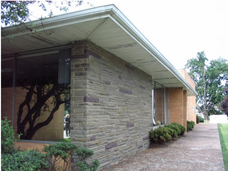
Plate 83. General Motors Corporation Training Center, Office, Façade (North Elevation), Looking Southwest.
