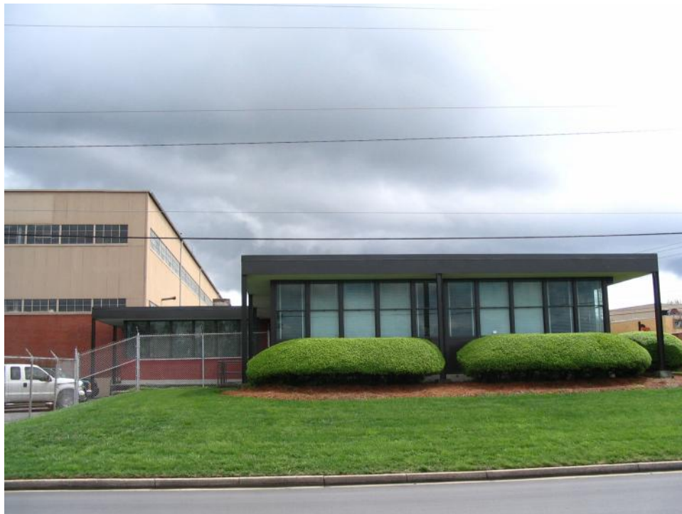
Plate 57. Republic Steel Corporation Plant, Office, North Elevation, Looking South.
