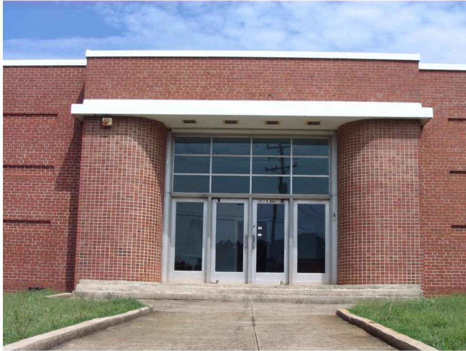
Plate 26. Chadbourn Hosiery Mills, East Elevation, Entrance Detail.
