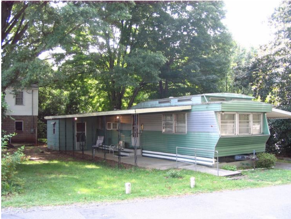
Plate 77. Elmore Trailer Sales and Trailer Park, Trailer Park, Looking Southeast.
