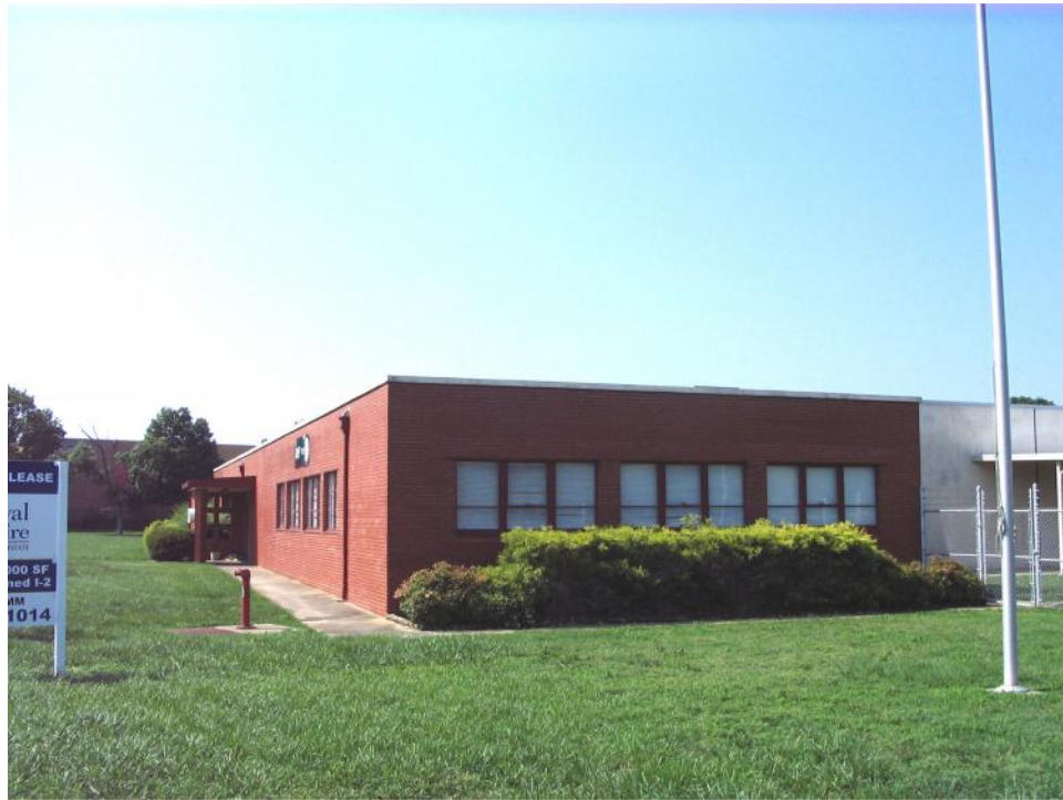
Kaiser Fluid Technologies Company Plant (No. 72), Side (North) Elevation.
