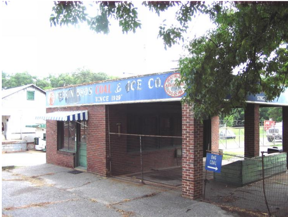
Plate 38. Herrin Brothers Coal and Ice Company Complex, Office, Looking Northeast.
