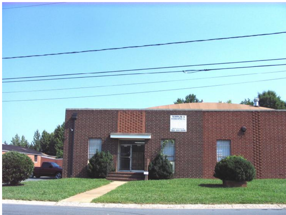
Industrial Building (No. 55).
