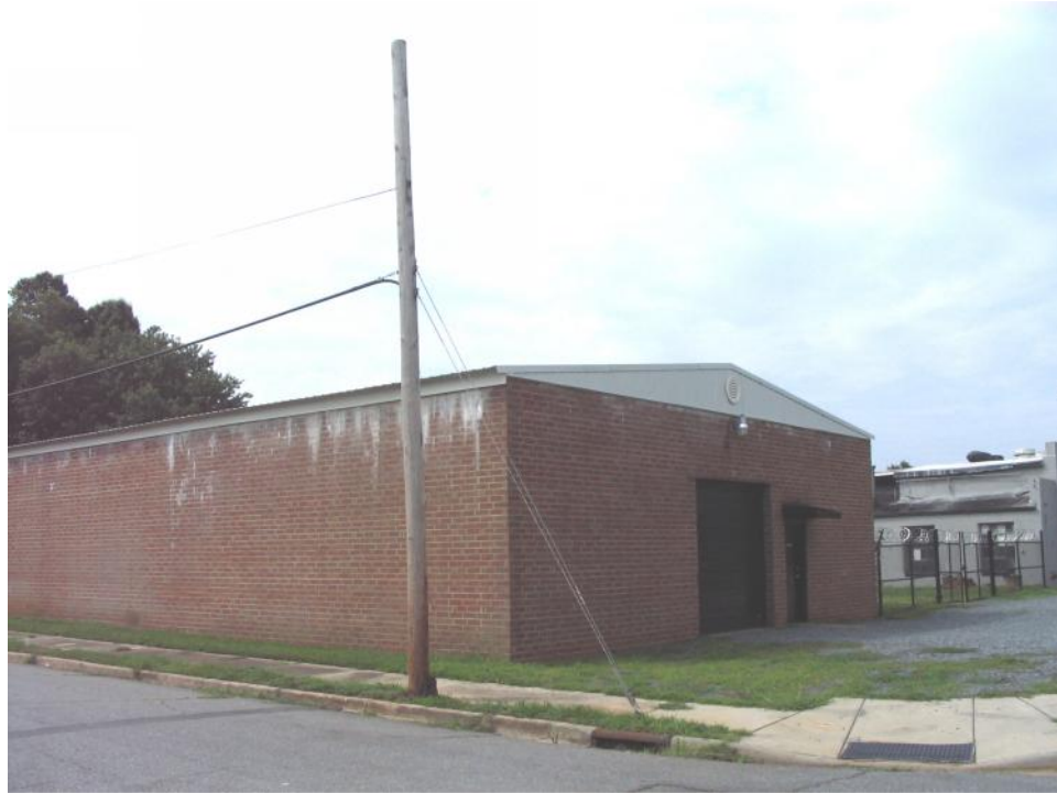
Machine Shop Complex (No. 18), 1960s Warehouse.
