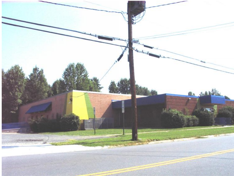
Industrial Building (No. 56).
