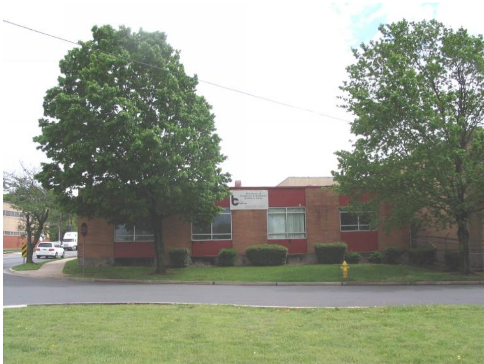
Plate 45. Standard Chemical Products Plant, Side (North) Elevation, Looking South.
