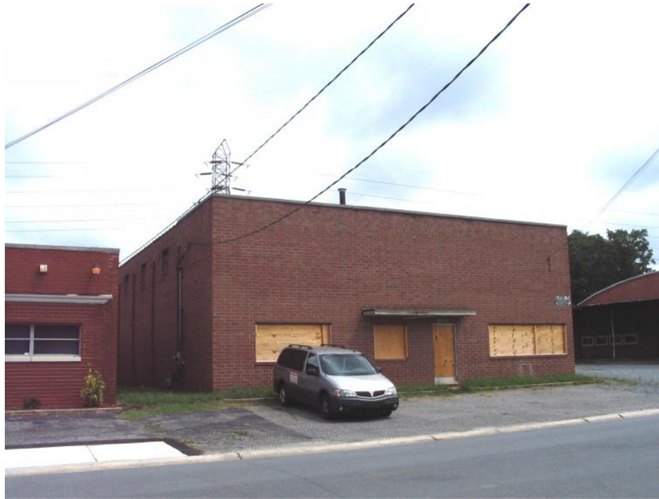
Industrial Building (No. 47).
