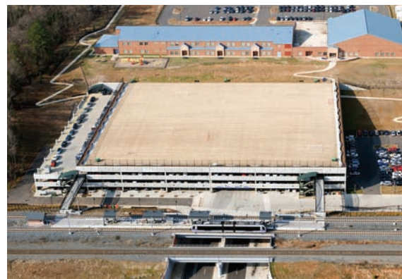
The LYNX I-485/South Boulevard parking deck.
