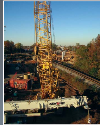
Installation of girders at Tyvola Road bridge
