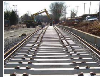
Railroad ties at Old Pineville Road
