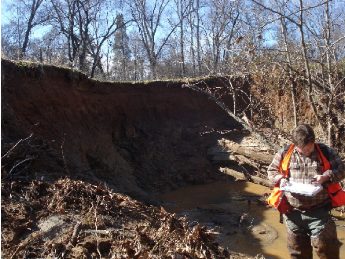
Figure 12: Severe Erosion along West Branch of the Rocky River.
