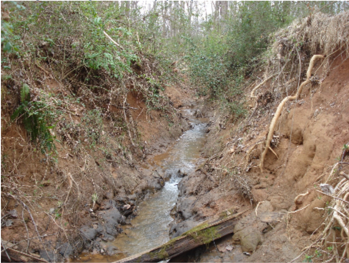
Figure 4: Straightened tributary of Rocky River.
