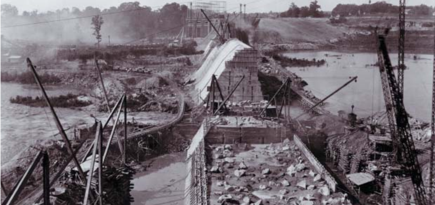
Construction of Mountain Island Dam, September 12, 1923.
