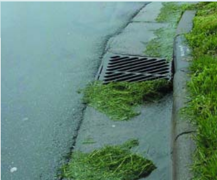
It is illegal to dump, blow or sweep grass clippings into storm drain.
