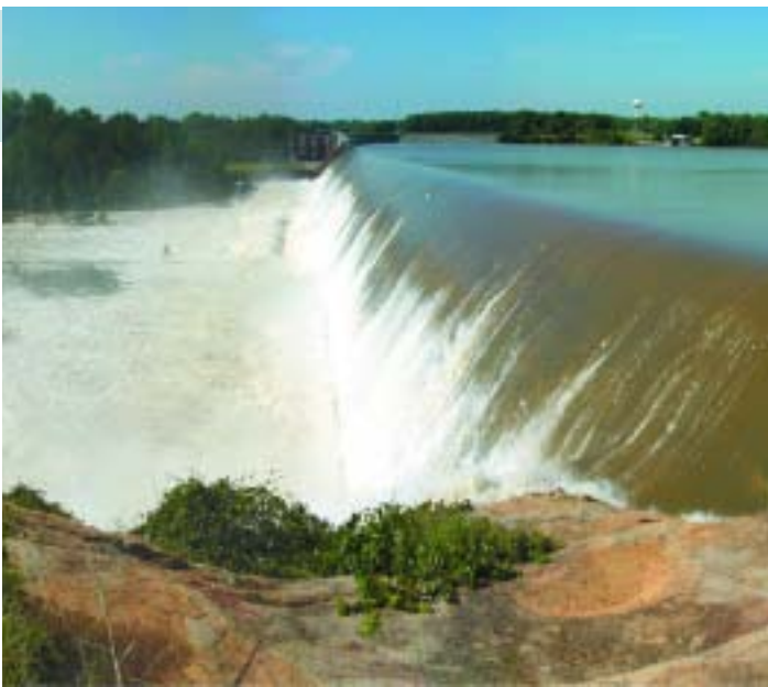
Water running over Mountain Island Dam following heavy rains in September 2004.
