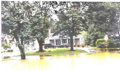
Home Built after Floodplain Regulations
