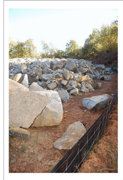
A contractor has piled 3,000 tons of boulders and rock in a field on Gilead Road. Frank DeLoache/Herald photo
