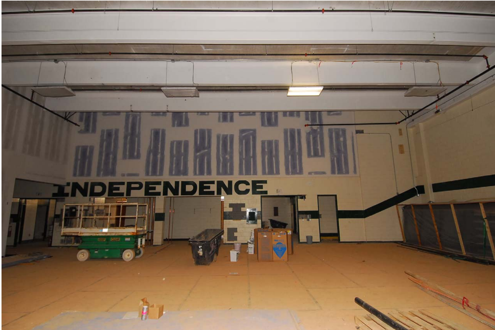
Independence High School New Gymnasium
