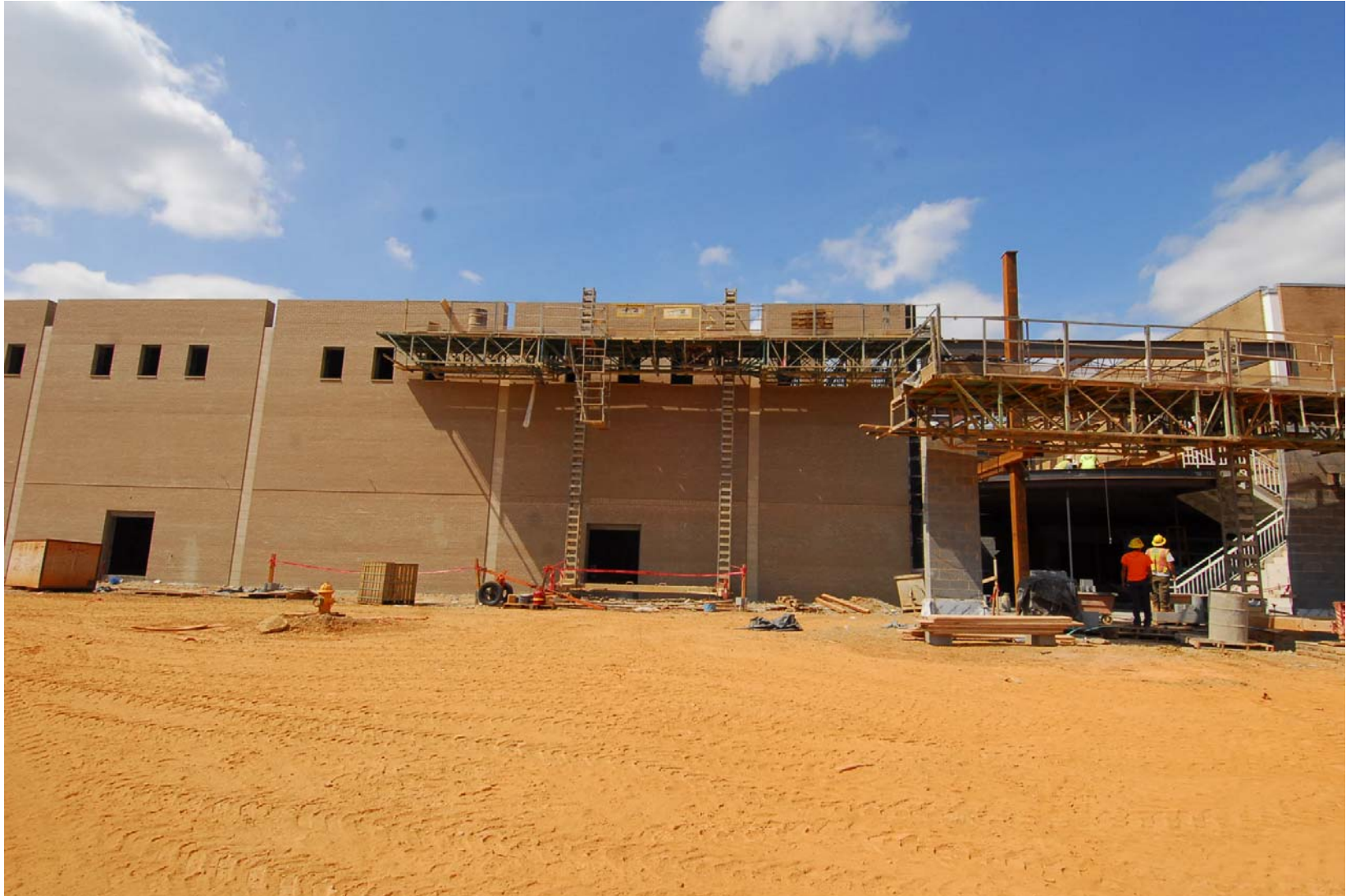
Independence High School New Gymnasium
