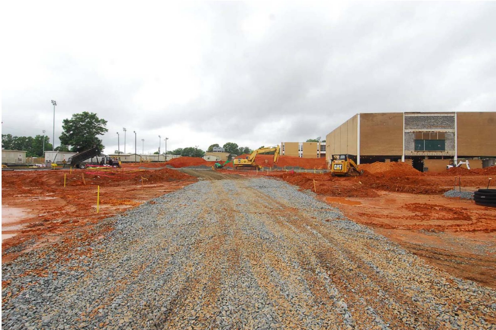
Independence High School New Gymnasium
