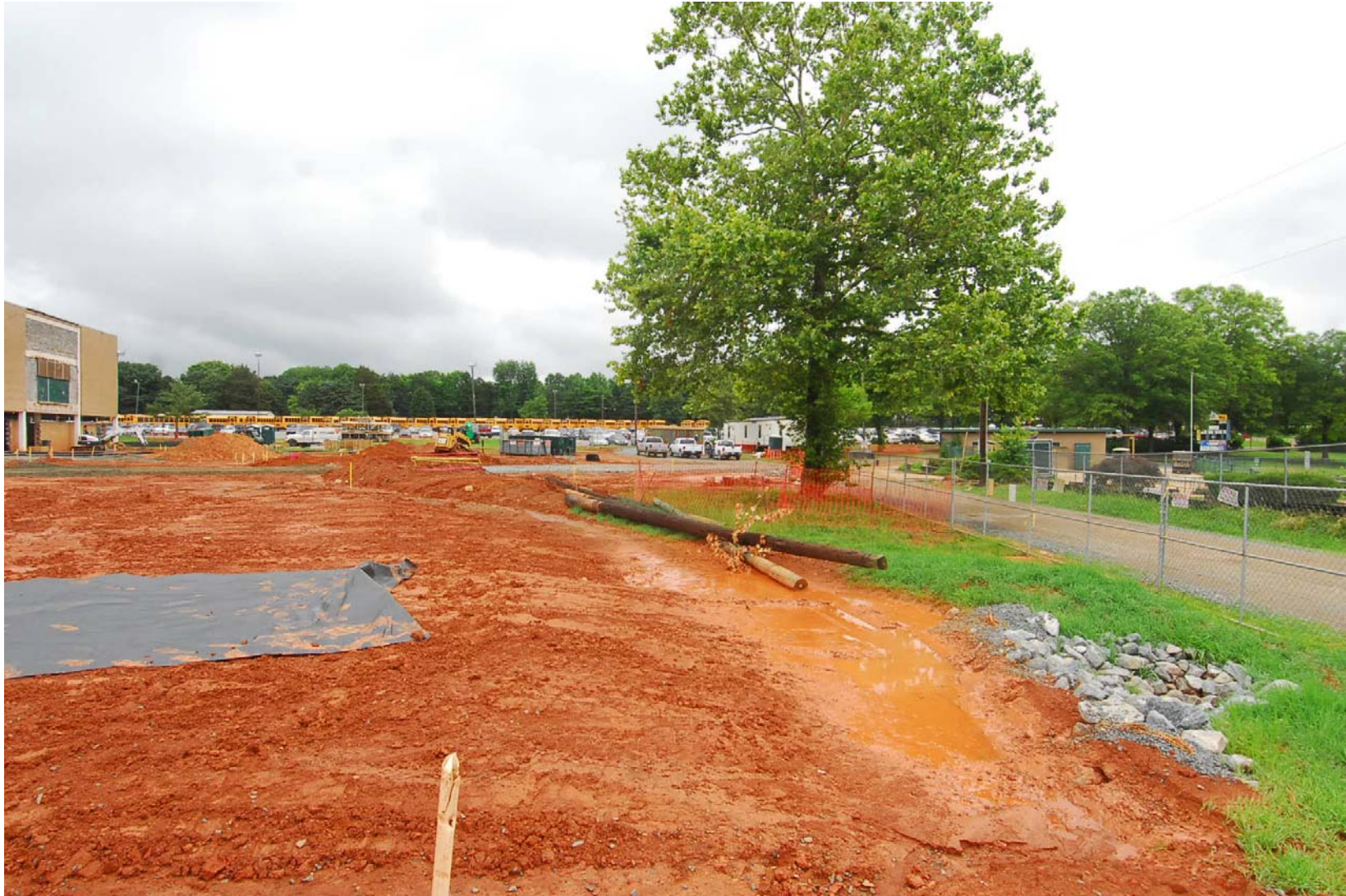
Independence High School New Gymnasium
