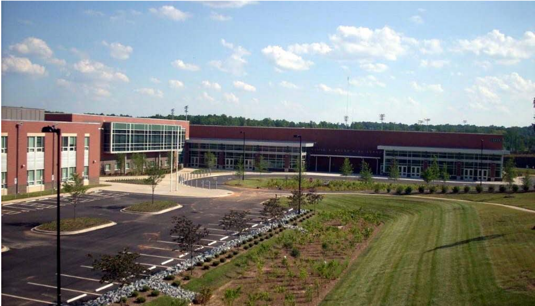
Hough High School (H07-02) Main Entrance
