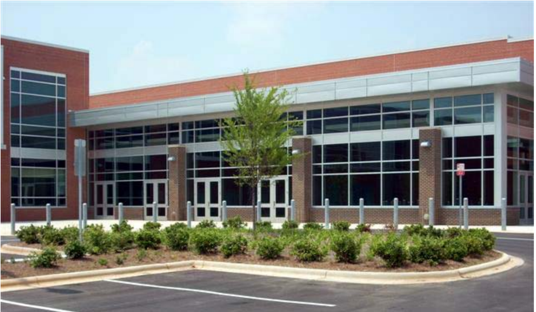
Rocky River High School (H07-01) Main Entrance
