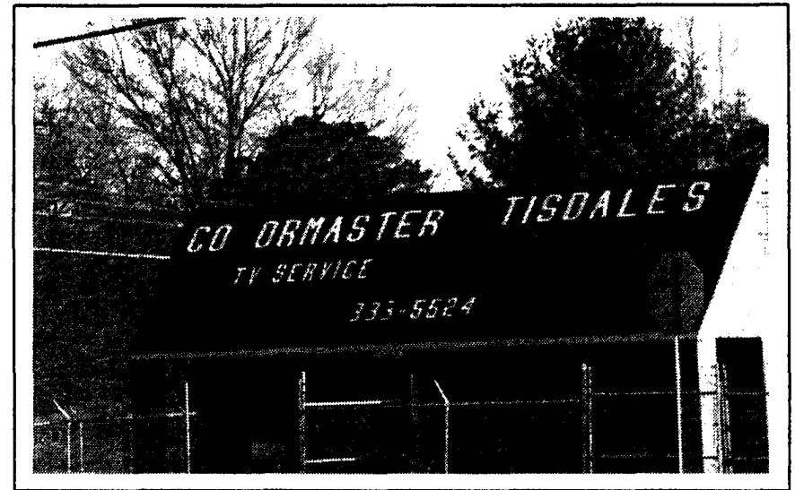
Poorly maintained signs should be cited for zoning code violation.
