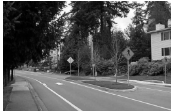
Pedestrian refuge medians are recommended along Hawthorne Lane in the vicinity of Sunnyside Avenue.
