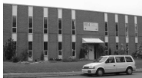
Metrolina Association for the Blind office building occupies Area 2.
