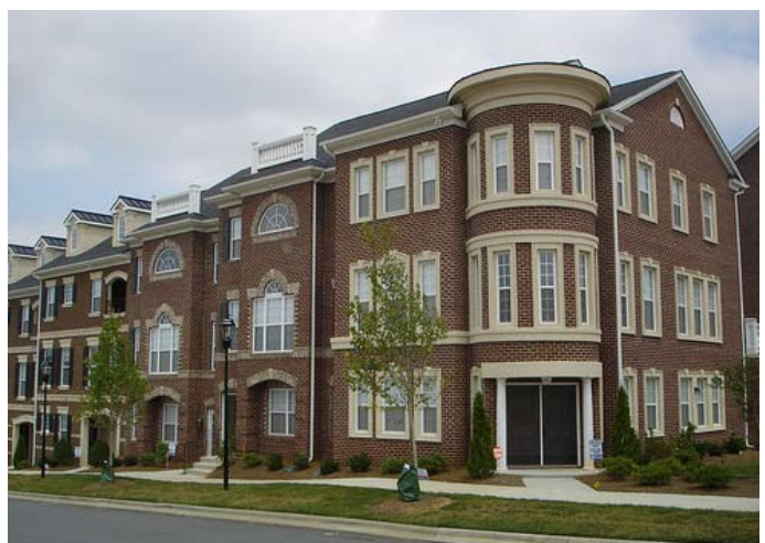
Ayrsley Town Center was one of the first mixed use developments in the area.
