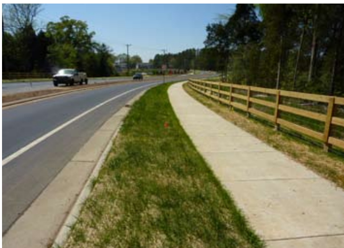
Shopton Road West near Steele Creek Road is an example of a newly improved thoroughfare, including new turn lanes, median islands, bicycle lanes, planting strips and sidewalks.
