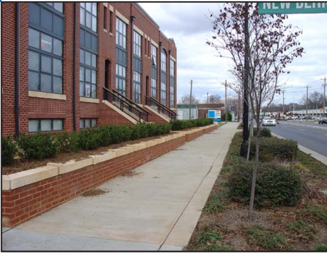
3030 South is an example of transit oriented development pushing south from South End.
