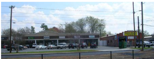
Existing commercial development tends to be auto oriented, suburban type design.
