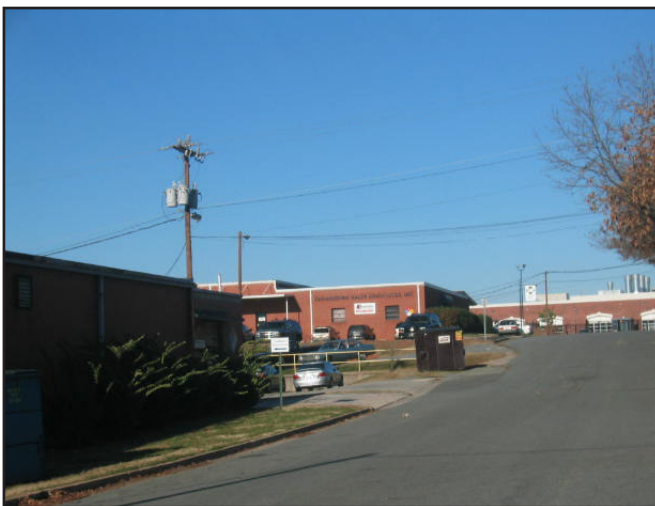
The Scaleybark area has a substantial stock of older warehouse and industrial properties where redevelopment might occur.
