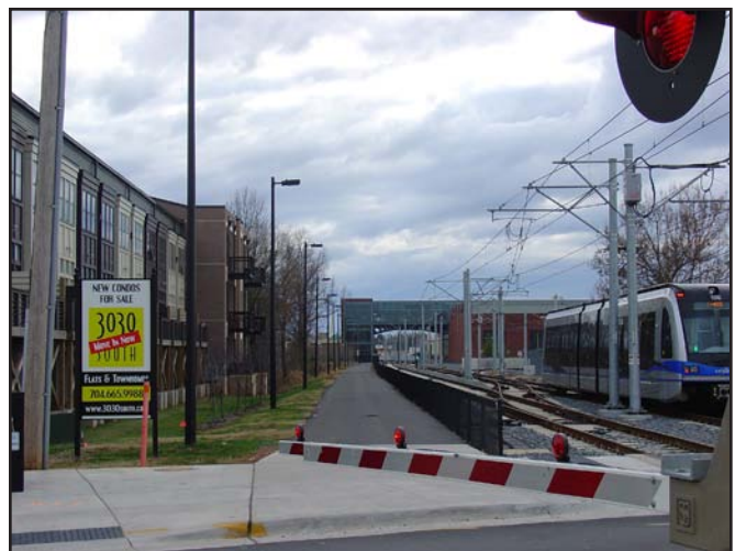
New residential development and multi-use trail near the New Bern station.
