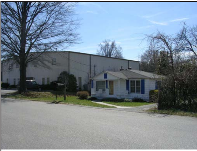
Residential and industrial uses adjoin in a number of places throughout the study area.
