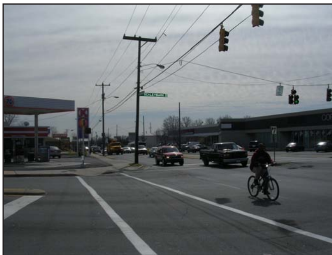
The pedestrian system along South Boulevard typically lacks a planting strip, and the sidewalk width is inadequate.
