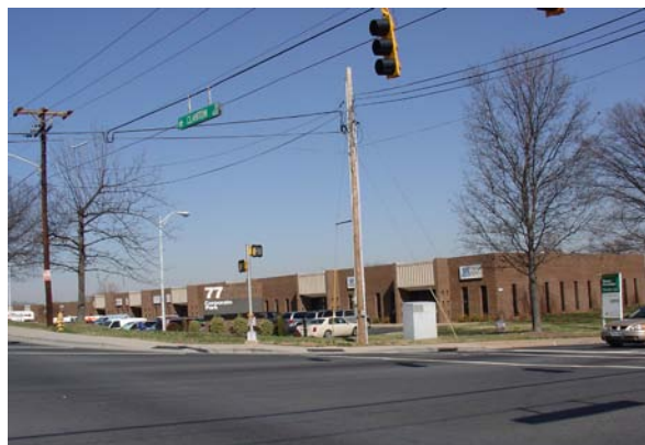
Existing industrial buildings in the station area are single story industrial park type properties.
