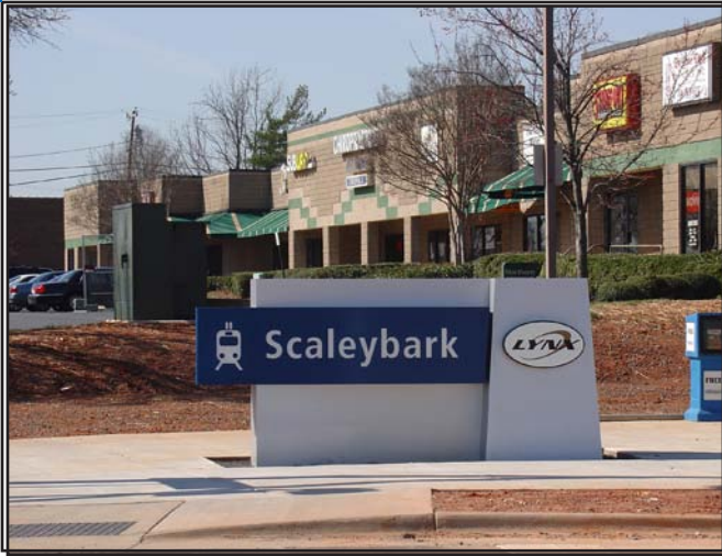
Properties adjacent to the Scaleybark Station are lower density uses ready for redevelopment..
