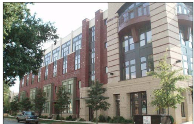
Higher density transit supportive development such as this is appropriate in the Transit Station Area.
