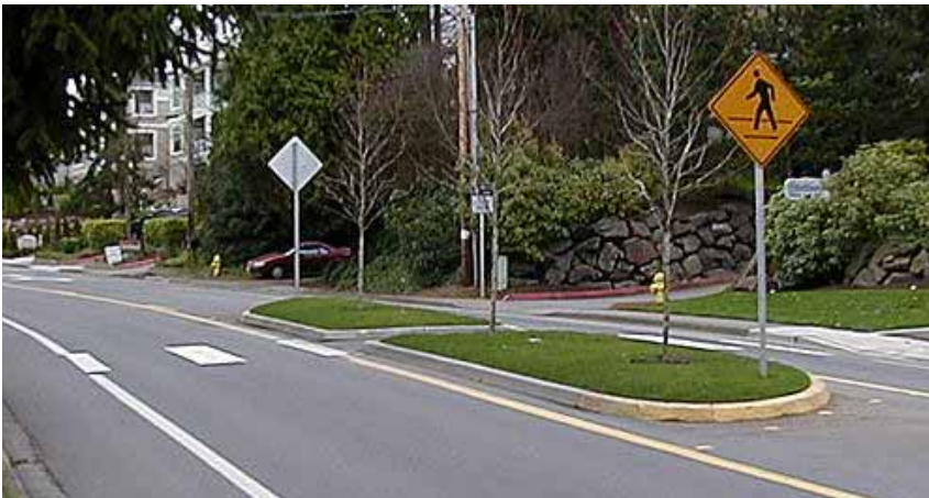
Example of a pedestrian refuge median
