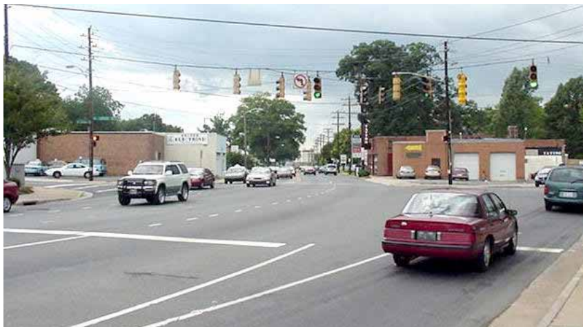
The Central Five Points intersection is a particularly difficult location for pedestrian crossings
