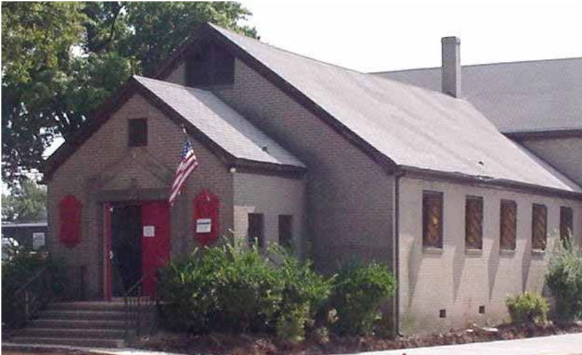
Former church rezoned MUDD-O for commercial reuse
