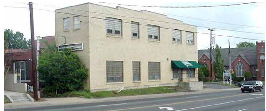
Existing buildings limit the ability to widen the street
