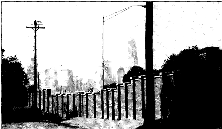
A sound barrier wall minimizes the impact of Independence Blvd. on adjacent neighborhoods.
