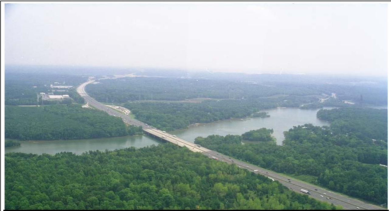
The I-85 Bridge crosses the pristine shoreline of the Catawba River, connecting Mecklenburg County to Gaston County.
