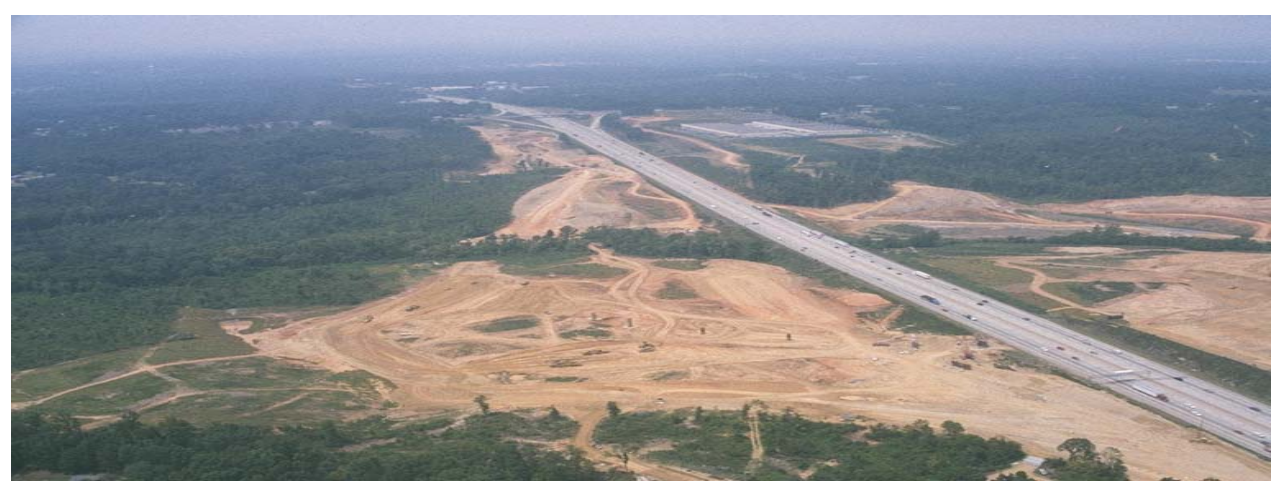
Location of future interchange of I-485 and I-85.
