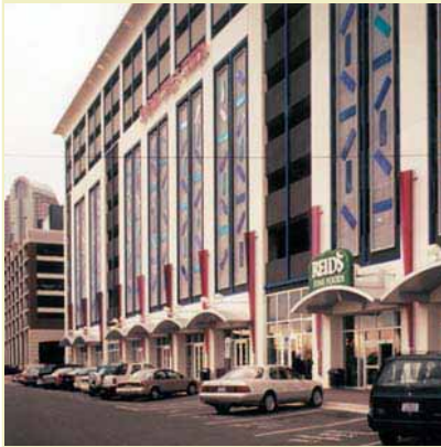
Figure 79: Center City has pursued innovative parking structure design, such as Seventh Street Station.
