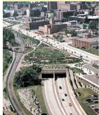
Figure 55: The highway cap in Duluth, Minnesota was originally constructed as a citywide park. Adjacent construction of a high-tech office complex has created a campus-like atmosphere.
