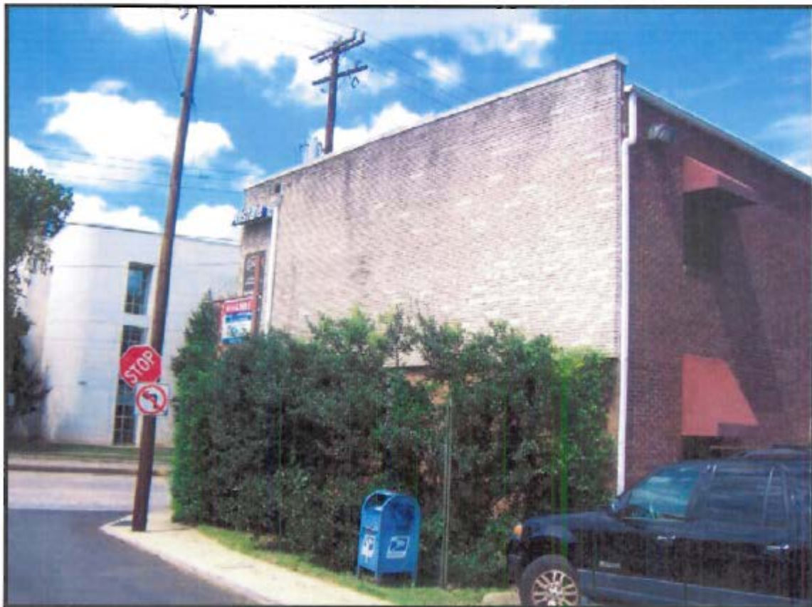
Side view of subject improvements taken from East 5 th Street.
