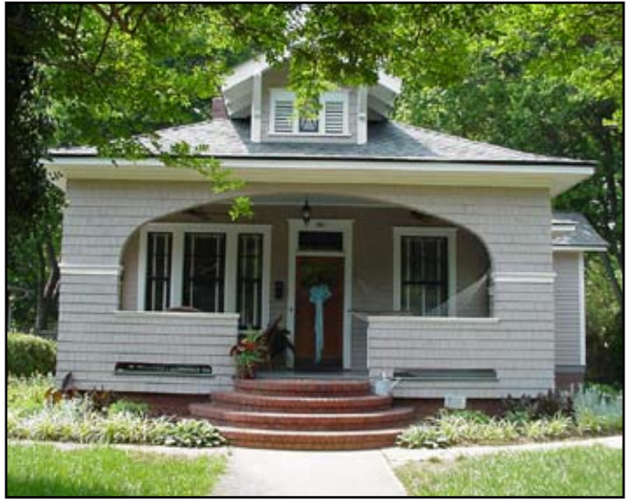
• The open porch was reestablished based on historic photographs of the house.
