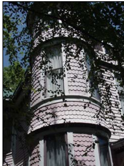
• Shingles create many different patterns and are often interchangeable with other appropriate forms of siding.
