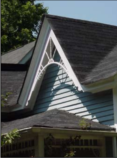
• Distinctive stick work is a detail appropriate only to the High Victorian style.
