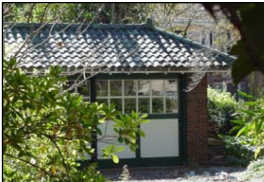
• Design and materials are derived from the main structure.
