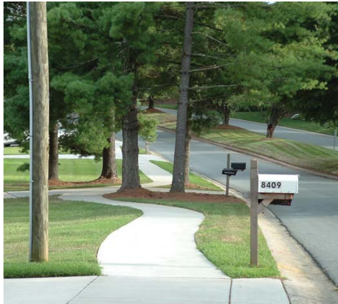
a new sidewalk in a subdivision
