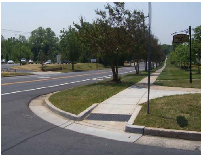
Charlotte continues to retrofit sidewalk with handicapped ramps.
