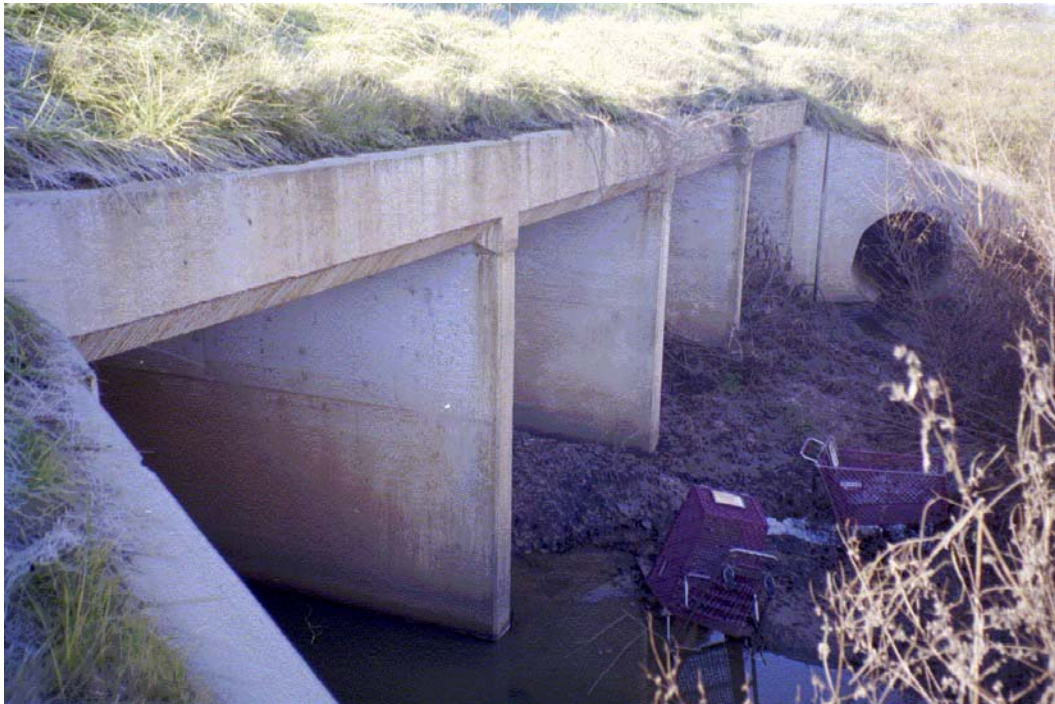
Coffey Creek View, U/S FACE
