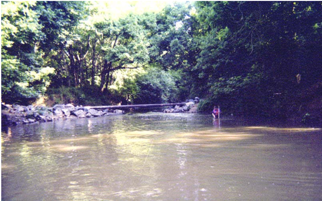
Sugar Creek View, D/S Roll #6 Photo #9 SUGAR CREEK BETWEEN ARROWOOD ROAD AND S. TRYON STREET. SANITARY SEWER CROSSING WITH POOL BELOW 4-6 FEET DEEP. LIVE CLAMS IN SAND.
