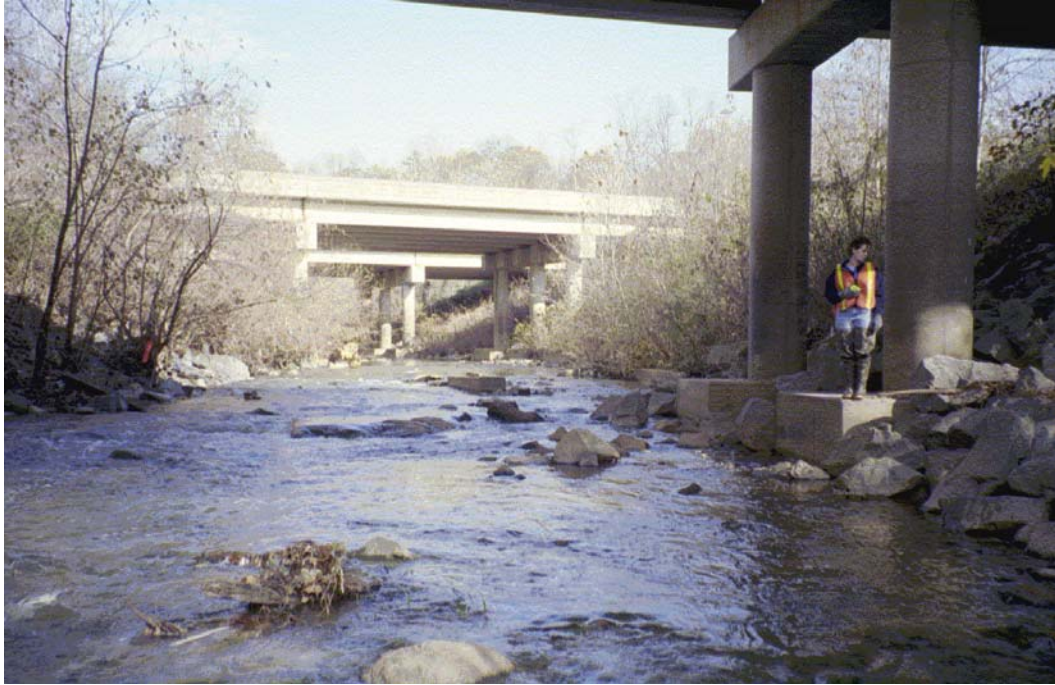
Sugar Creek View, D/S FACE Roll #2 Photo #14 UNDER YORKMONT ROAD BRIDGE. DOWNSTREAM FACE OF BILLY GRAHAM PARKWAY BRIDGES IN DISTANCE. BOTTOM MATERIAL IS COBBLES AND BOULDERS. VEGETATION PROTECTS BANKS.
