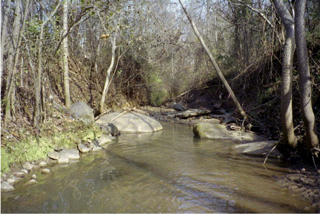
Kings Branch View, U/S Roll #2 Photo #9 LOOKING UPSTREAM OF HEBRON STREET. STREAM DOWNCUTTING WITH STEEP, SEVERLY ERODED BANKS. BOULDERS PRESENT IN CHANNEL.
