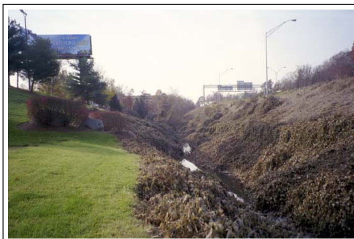
Figure 10. Kings Branch Along I-77 Corridor, Facing Downstream (Roll #2, Photo #2)
