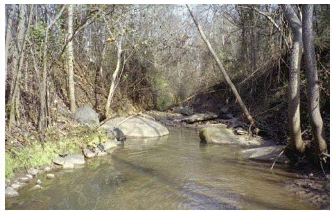
Figure 3. Typical Channel, Kings Branch Looking Upstream of Hebron Street (Roll #2, Photo #2)
