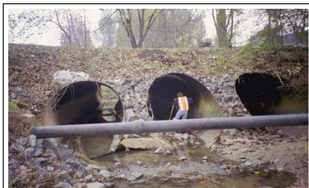
Figure 6. Sanitary Sewer Crossing at Kings Branch Below Archdale Road (Roll #1, Photo #22)
