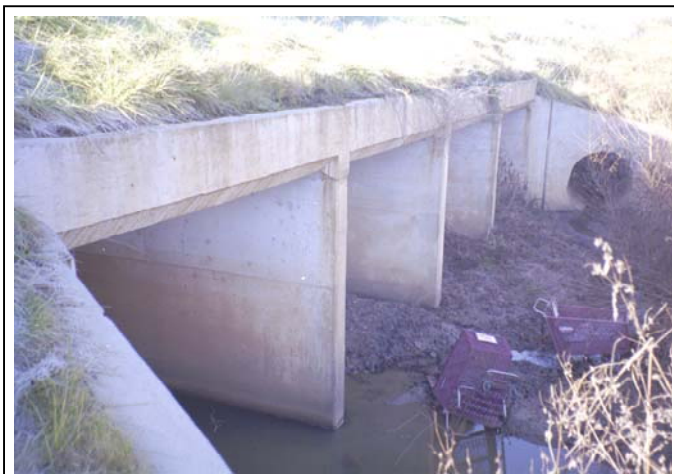
Figure 8. Heavy Sedimentation and Debris on Coffey Creek at Arrowood Drive (Roll #1, Photo #14)
