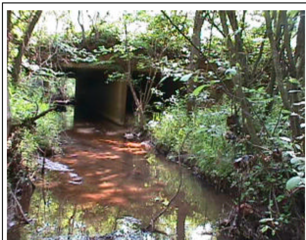
Fig. 5 Caldwell Station Creek at Statesville Road
