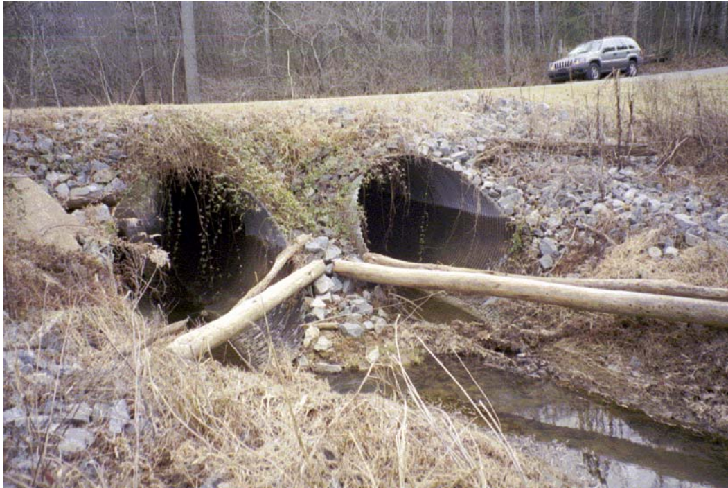
Stoney Creek Tributary View U/S Roll #2 Photo #14 DEBRIS BLOCKING UPSTREAM FACE OF 2 BARREL 6'8" CMP CROSSING AT HOMEWOOD DRIVE.
