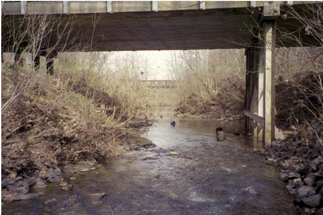
Mallard Creek View, D/S Roll #2 Photo #6 BRIDGE CROSSING AT MALLARD CREEK CHURCH ROAD. PEDESTRIAN BRIDGE AND NCDOT MITIGATION WETLAND PRESENT IN BACKGROUND.
