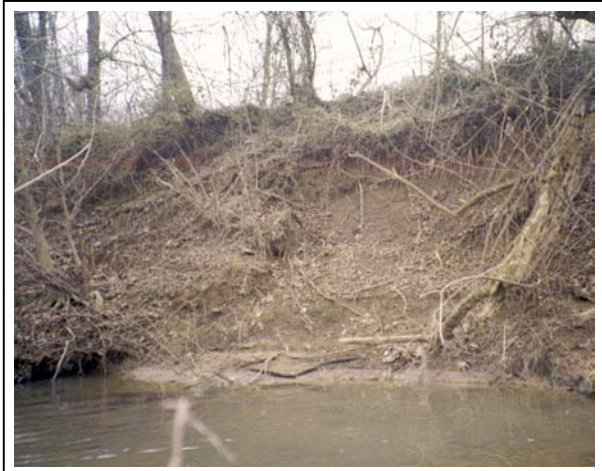
Figure 17. Bank Erosion, Mallard Creek Looking Downstream of I-85 (Roll #2, Photo #1)
