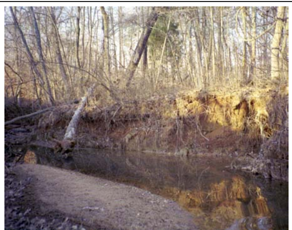
Figure 16. Bank Erosion, Doby Creek Upstream of Governors Road (Roll #2, Photo #22)
