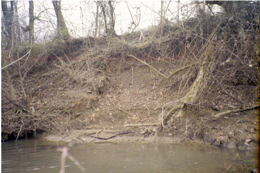
Mallard Creek View, D/S Roll #2 Photo #1 EXTENSIVE RIGHT BANK EROSION NEAR I-85 CROSSING. EXPOSED ROOTS AND TREE COLLAPSED.
