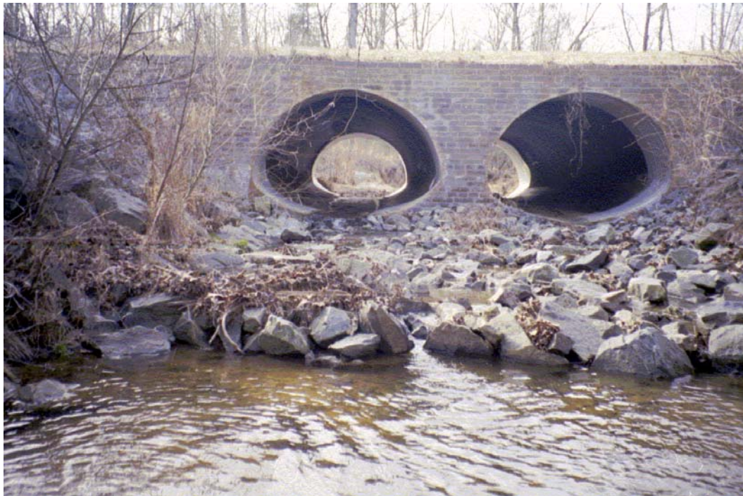
Toby Creek View D/S Roll #3 Photo #12 DROPOFF AT DOWNSTREAM FACE OF 2 BARREL 12' x 18' CMPA ROCKY RIVER ROAD CROSSING.
