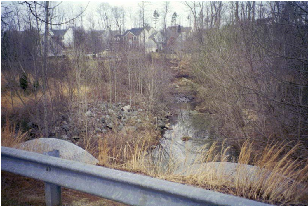
Clarks Creek View, U/S Roll # DEVELOPMENT UPSTREAM OF SAXONBURY WAY CROSSING.
