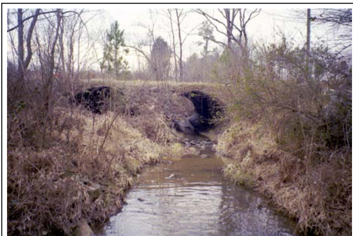
Figure 2. Typical Channel, Clarks Creek at Dearmon Road, Downstream Face (Roll #1, Photo #2)
