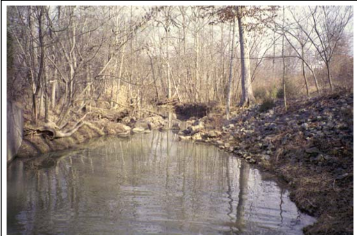
Figure 6. Typical Channel, Stoney Creek near I-85, Looking Downstream (Roll #2, Photo #12)
