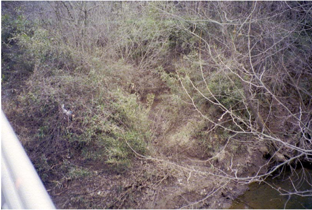
Mallard Creek View, U/S Roll #2 Photo #8 TRIBUTARY EROSION AND DOWNCUTTING IN RIGHT BANK NEAR PAVILION ROAD BRIDGE CROSSING.
