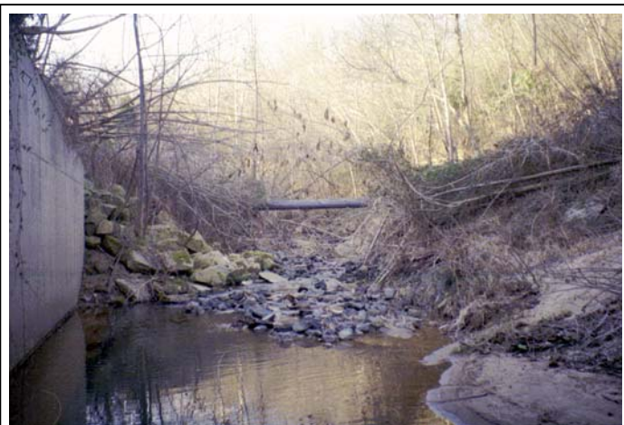
Figure 4. Typical Channel, Doby Creek Upstream of W.T. Harris Boulevard (Roll #2, Photo #23)
