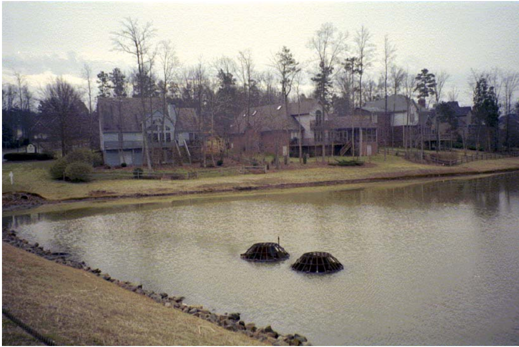
Clarks Creek Tributary #1A INTAKE STRUCTURES AT DAVIS LAKE.
