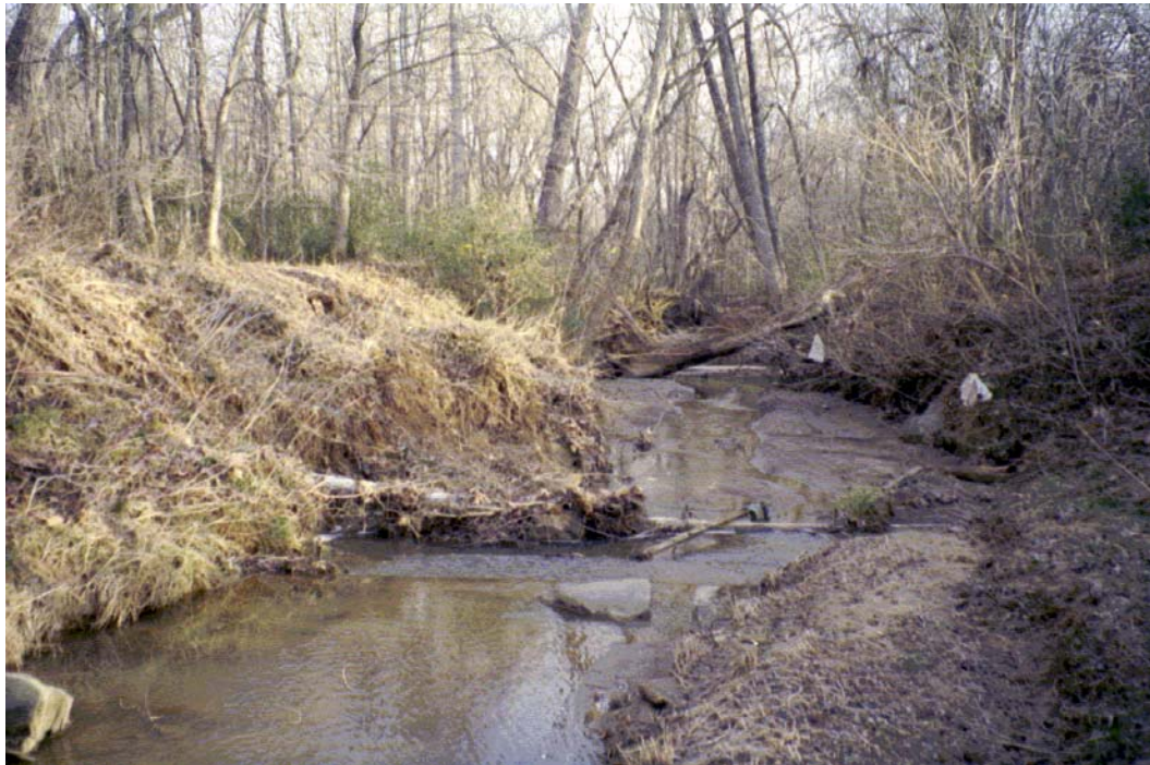
Toby Creek View D/S Roll #3 Photo #4 GRADE CONTROL IN FORM OF 2 WOOD PLANKS PRESENT DOWNSTREAM OF CONCRETE BOX CULVERT CROSSING AT RAMP TO WEST HARRIS BLVD FROM UNIVERSITY CITY BLVD SOUTH.
