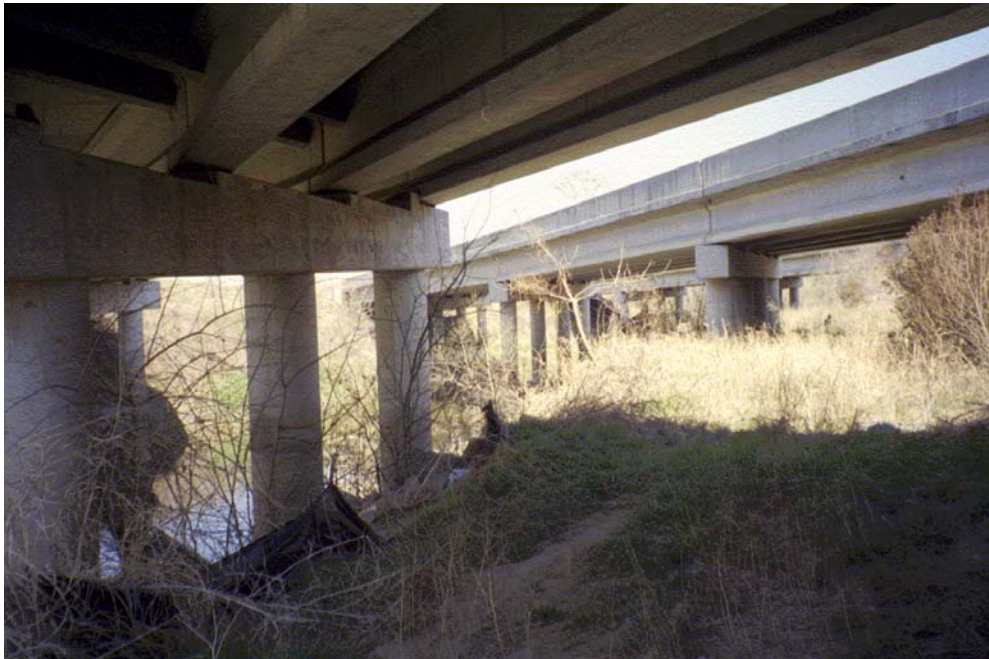
Lower Little Sugar Creek View (under bridge) Roll #4 Photo #16 I-485 THREE BRIDGE CROSSING (WEST BOUND, EAST BOUND, AND EAST BOUND RAMP).
