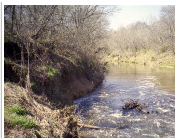
Figure 10. Erosion, Lower Little Sugar Creek at Polk Road, Looking Downstream (Roll #4, Photo #21)
