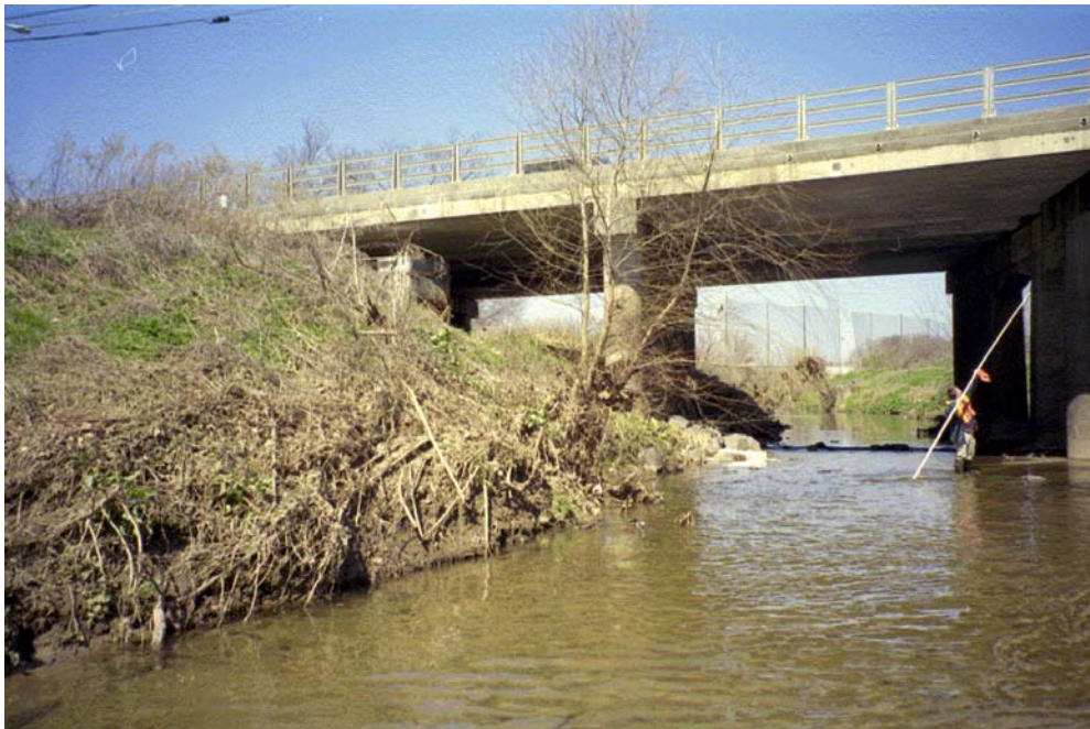
Lower Little Sugar Creek View D/S Roll #4 Photo #18 DOWNSTREAM FACE OF BRIDGE CROSSING HIGHWAY 51 (PINEVILLE-MATTHEWS ROAD).
