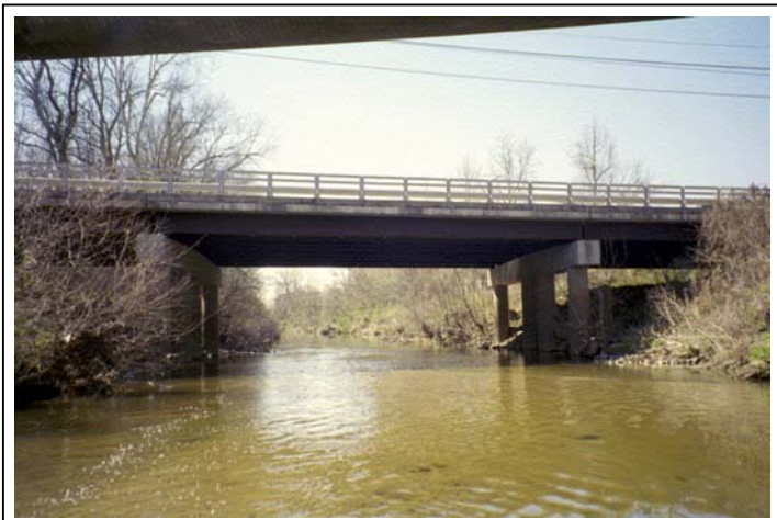
Figure 9. Realignment, Lower Little Sugar Creek at Sharon Road West (Roll #4, Photo #14)
