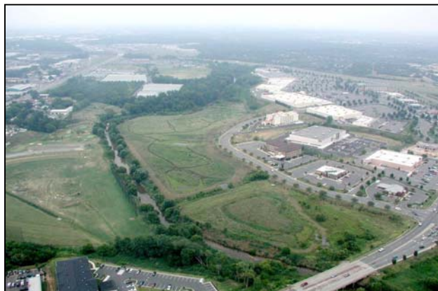
Figure 5. NCDOT Constructed Wetland at upstream of NC 51 (Photo Courtesy of MCSWS)
