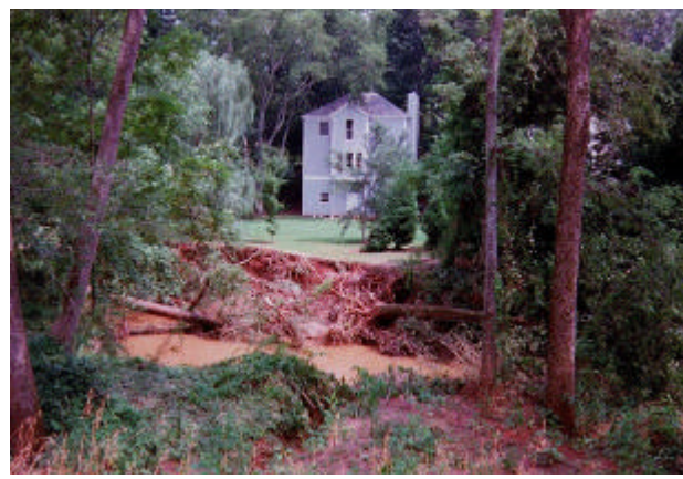
Figure 2. Briar Creek – Moncure Drive area before stabilization (provided by MCSWS).
