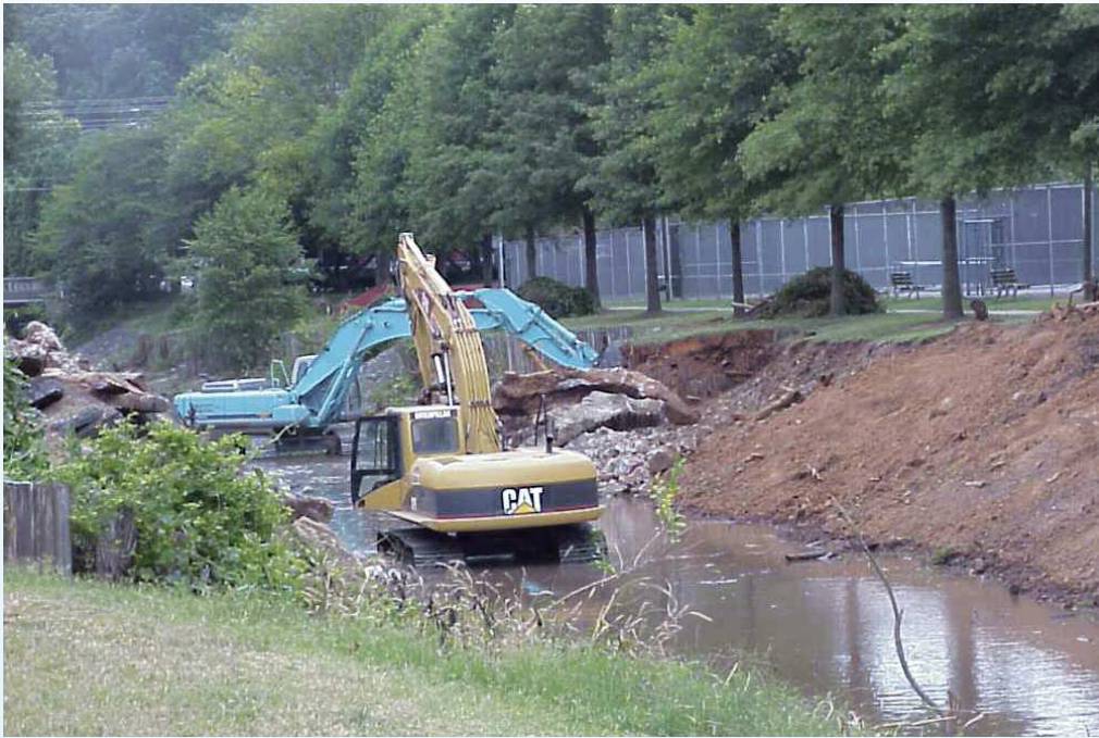
Stream restoration in Freedom Park.
