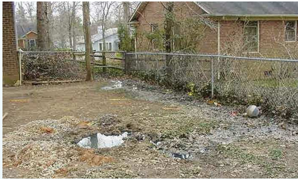
System failure: sewage surfacing on the ground and running along the property line.
