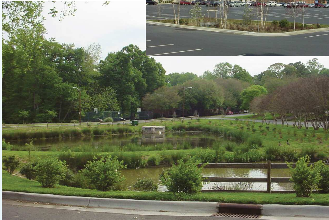
top New developments use bioretention areas, or “rain gardens,” to detain, clean, and slowly release runoff. The result is cleaner water and reduced flood risks. above This publicly funded retrofit in Charlotte is an attractive amenity that helps reduce water pollution.
