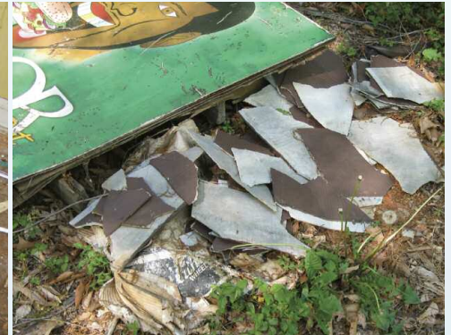
Asbestos-containing exterior siding removed during a renovation
