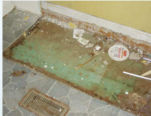
Green linoleum asbestos-containing floor tiles
