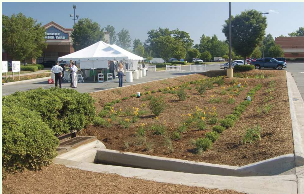
New rain gardens in Northcross Shopping Center in Huntersville, completed May 2008.
