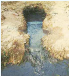
Discharge of raw sewage to Little Sugar Creek in 1972
