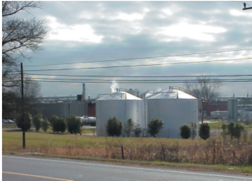
Typical polyurethane foam manufacturing facility.
