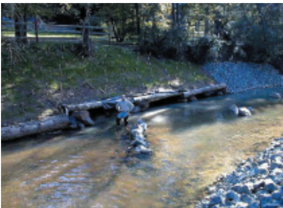
Fish lunkers, or constructed bank overhangs, installed in Briar Creek provide cover and refuge for fish.
