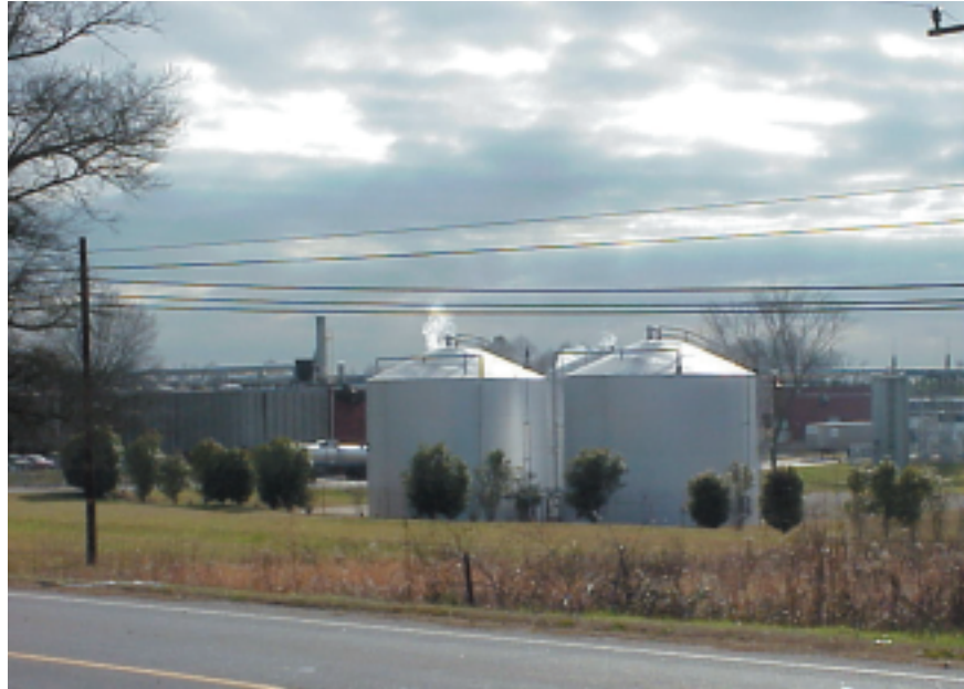
Typical polyurethane foam manufacturing facility.
