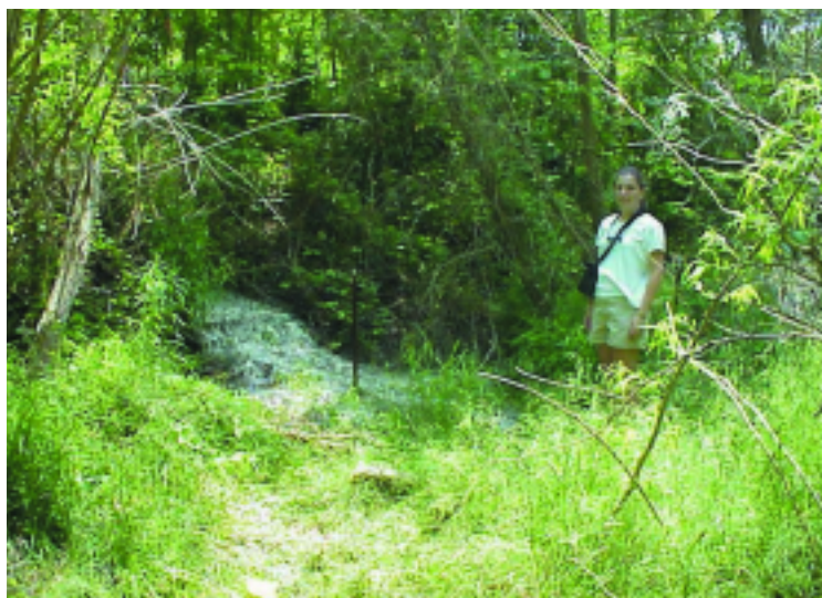
Leachate discharge (light colored liquid) at a closed landfill. Leachate is formed by water percolating through waste.
