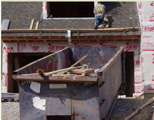
Photo 6.3 Residential Construction and Demolition Debris
