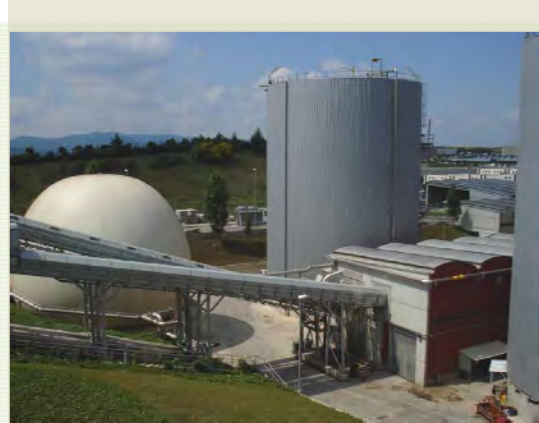
Photo 7.3 Anaerobic Digestion Facility in Spain
