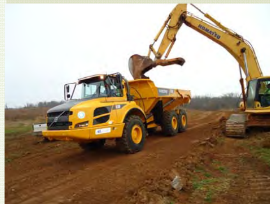
Photo 7.1 New Equipment at Foxhole Landfill
