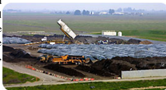
San Francisco Compost Facility
