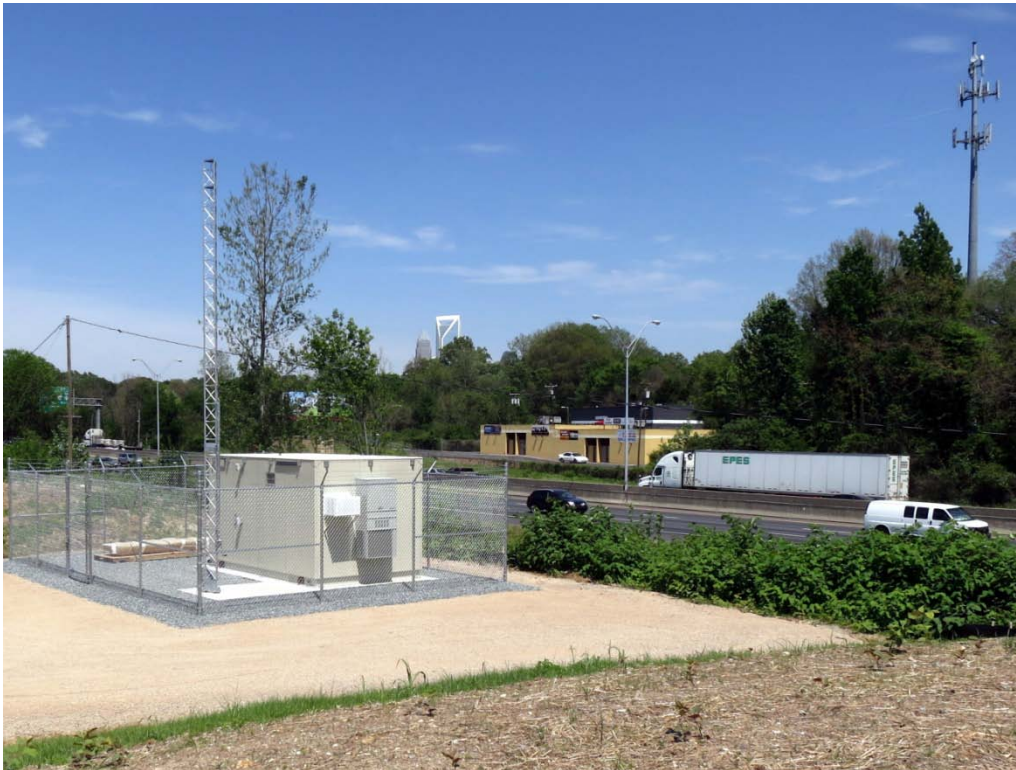
Figure 12. View of site toward roadway (I-77) looking NE with uptown Charlotte over the horizon.
