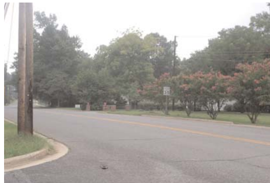
EXISTING CONDITIONS Photo of intersection at Main Street and Old Statesville Road, site of future roundabout
