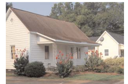
EXISTING CONDITIONS Photo of housing stock in Abernathy Park
