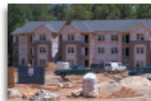
Construction at Tyvola Crossing is nearing completion.
