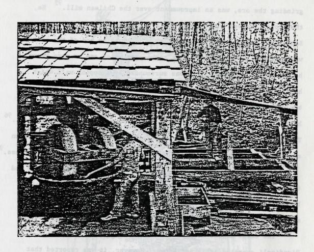
Figure 10. A Chilean mill and associated rockers of the type used at the St. Catherine mill (Photo taken at a mine near Salisbury, Rowan County about 1895)
