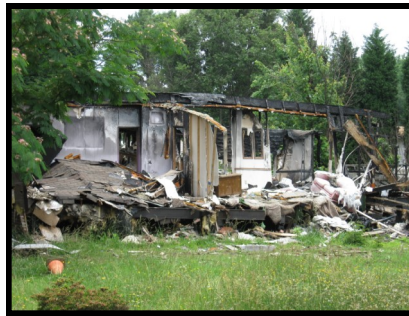
Environmental case is pictured prior to clean-up.
