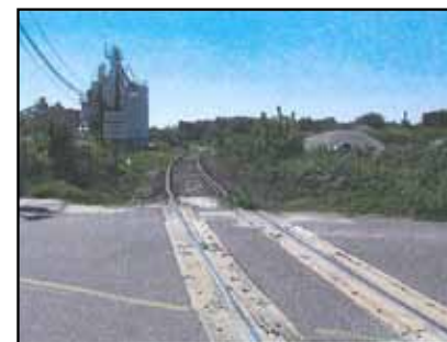
P&N Railroad Line with Concrete Plant in background (Gastonia, NC)
