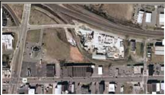
Future Site of Multi-Modal Transportation Center
