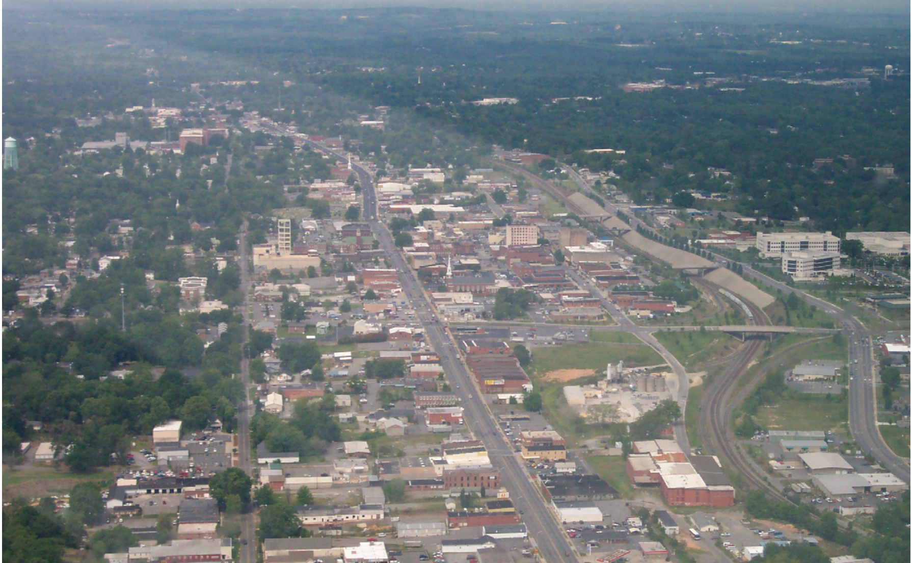
Aerial view of Franklin Boulevard, looking west, towards downtown Gastonia
