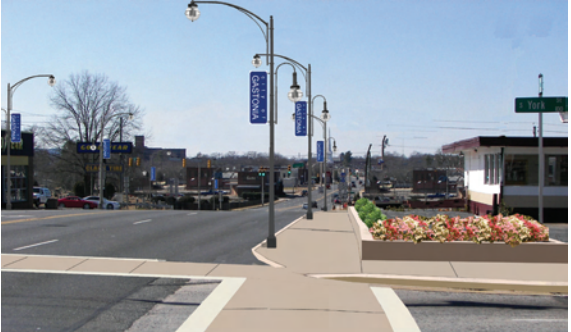
New crosswalks, curbs, flower beds + street lighting
