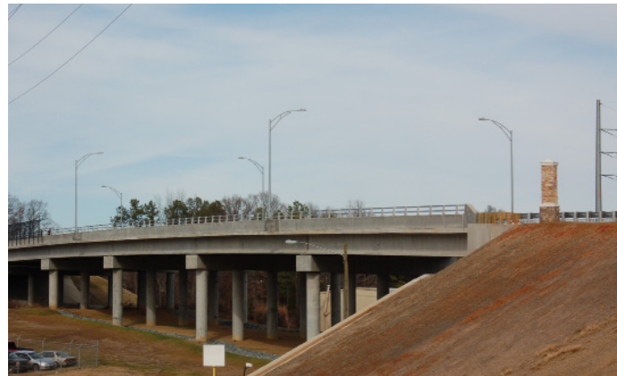
Built with concrete, the Fred D. Alexander Boulevard Project is Charlotte's first "green road." Currently under construction, it includes three bridges.
