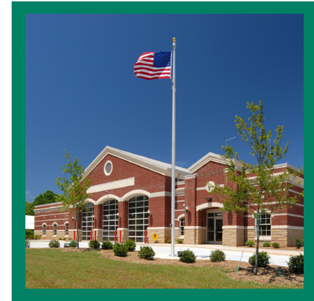
Completed in 2007, Fire Station 37 provides fire protection services for the south Steele Creek Area.
