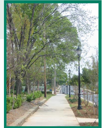
Charlotte residents have safe, convenient access to the LYNX Blue Line with the successful completion of the South Corridor Infrastructure Program.
